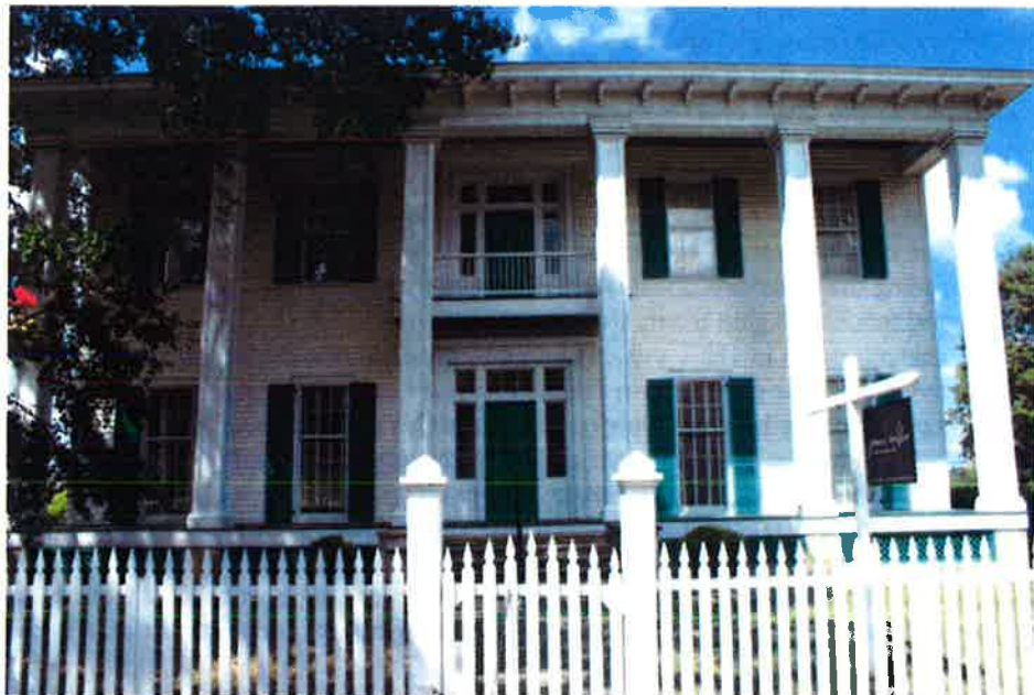
434 North McDonough Street
