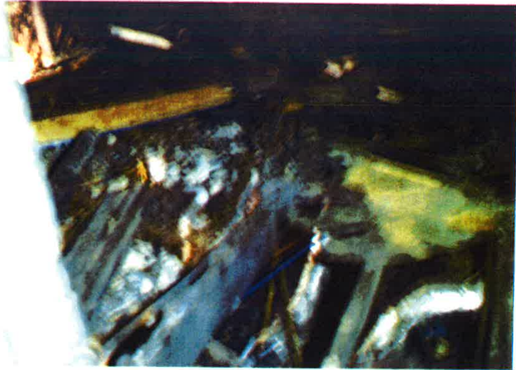
Second View of Floor Joists with Alligating Fire Damage of Joists
