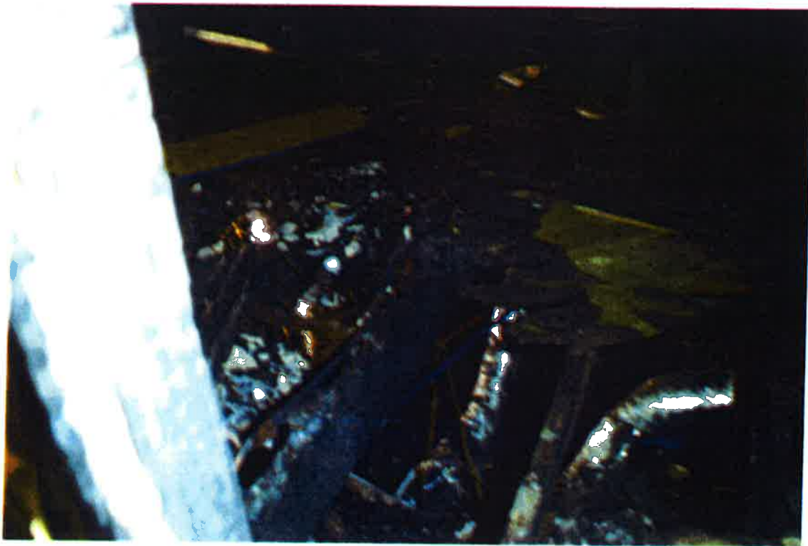
Second View of Floor Joists with Alligating Fire Damage of Joists
