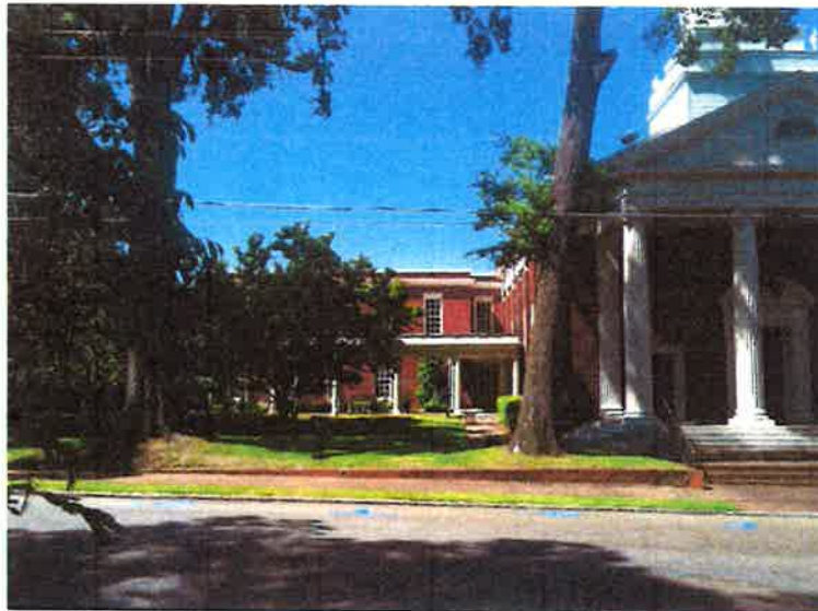
View of Location for New Handicap Ramp
