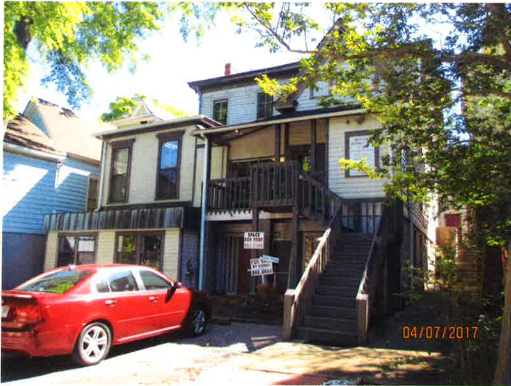
Decking on adjacent Sisters House
