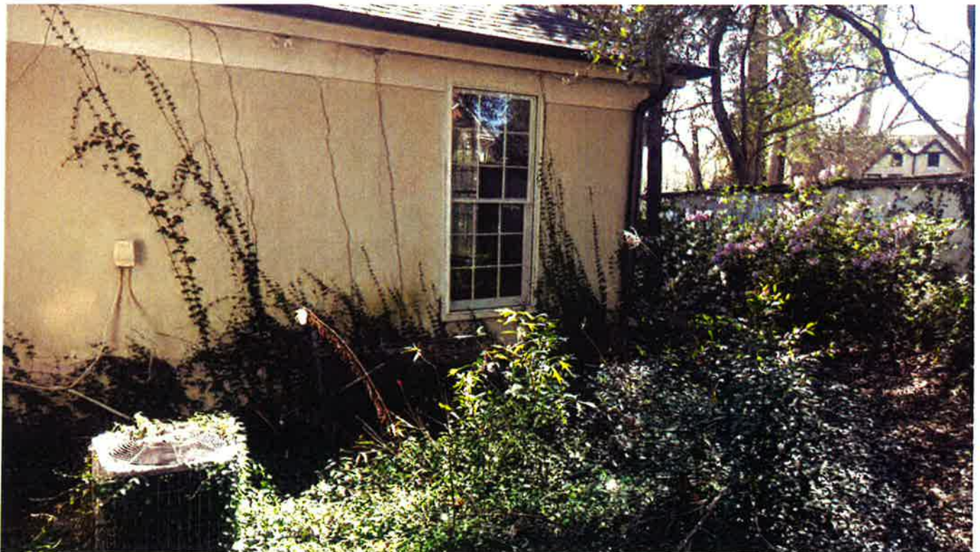
Rear of house looking south toward Cottage Place (behind wall)
