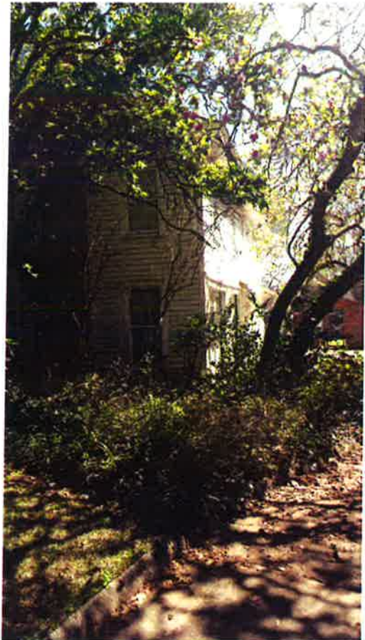
Southwest corner of subject structure, looking easterly
