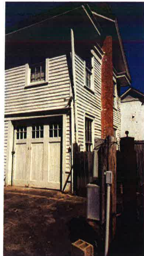
Southeast corner of subject structure, looking northerly
