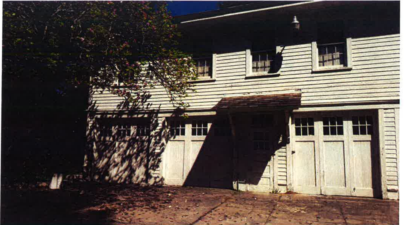
Front (south) side of structure, looking north
