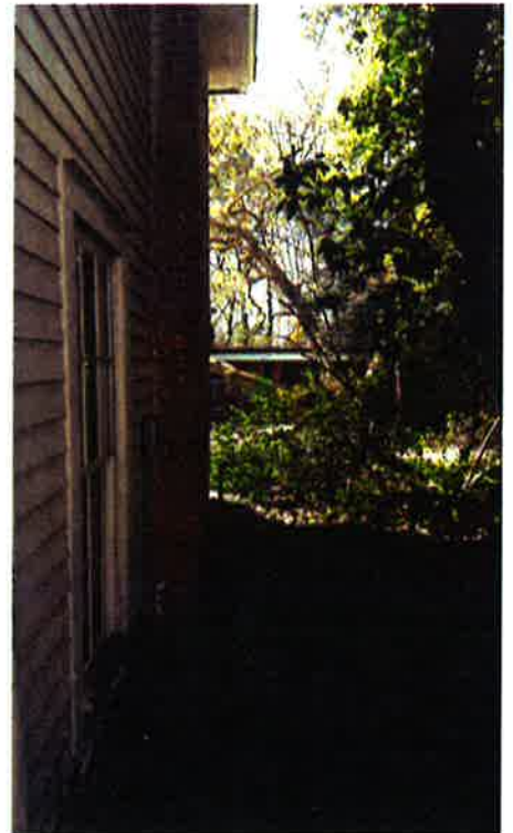
West side of subject structure looking south
