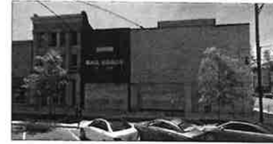
100 DEXTER AVENUE (CURRENT CONDITIONS)
