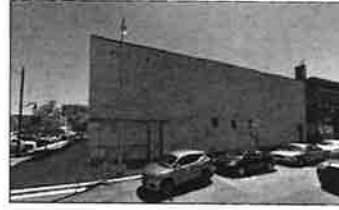
100 DEXTER AVENUE (CURRENT CONDITIONS)
