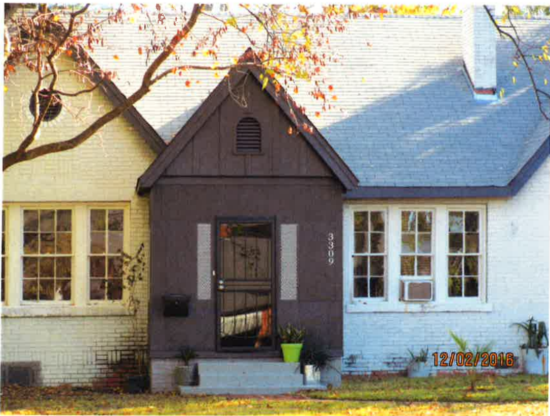
3309 Norman Bridge Road
