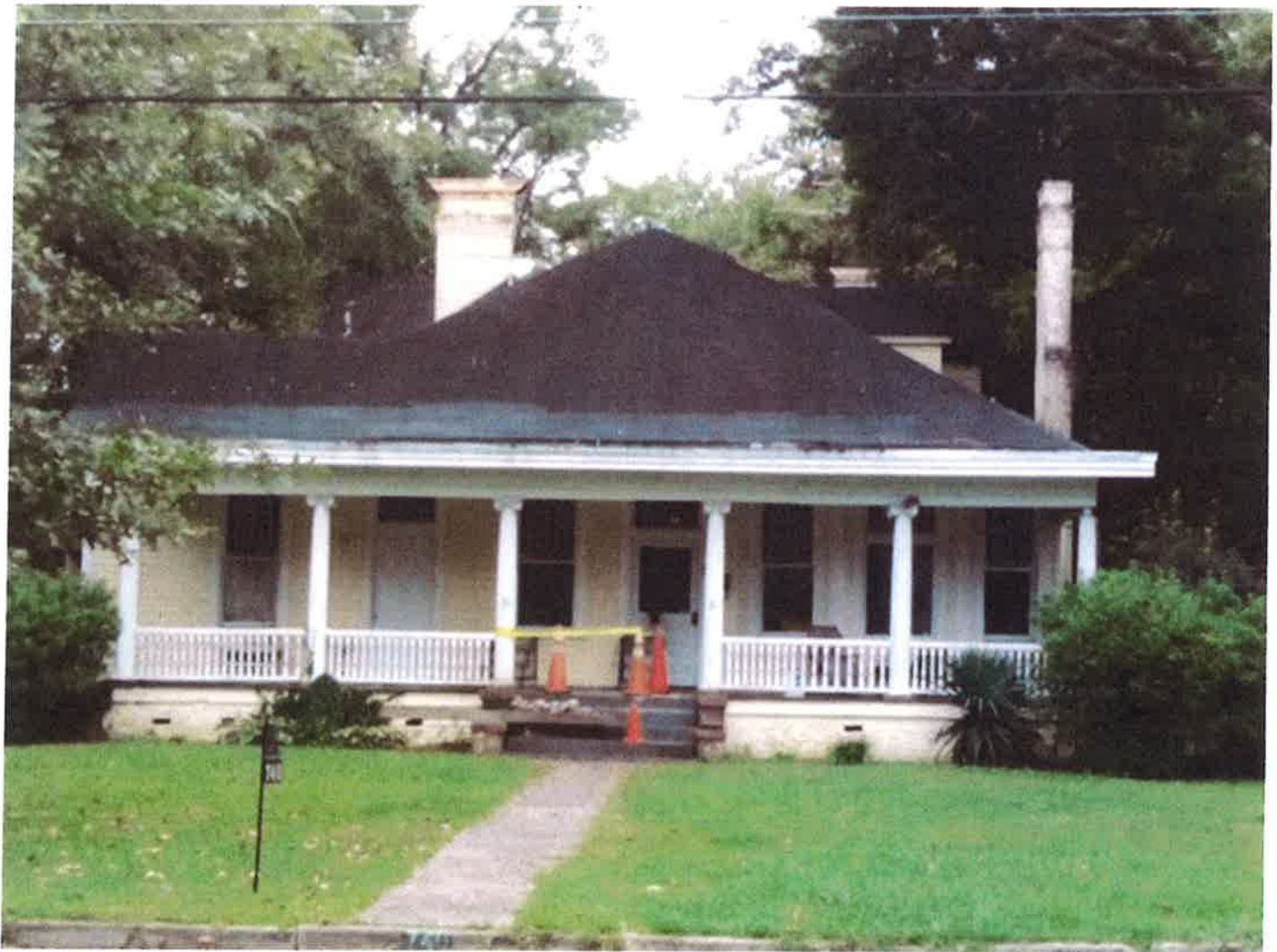
740 Felder Avenue Montgomery, Alabama (notice fluted Ionic columns & windows with diamond motif)
