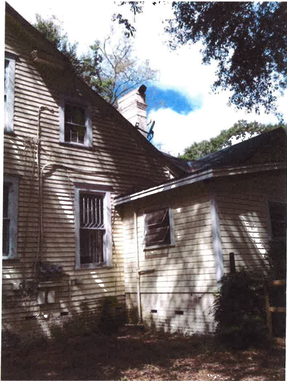
Left side (notice window w/ diamond motif to be moved to front of home)
