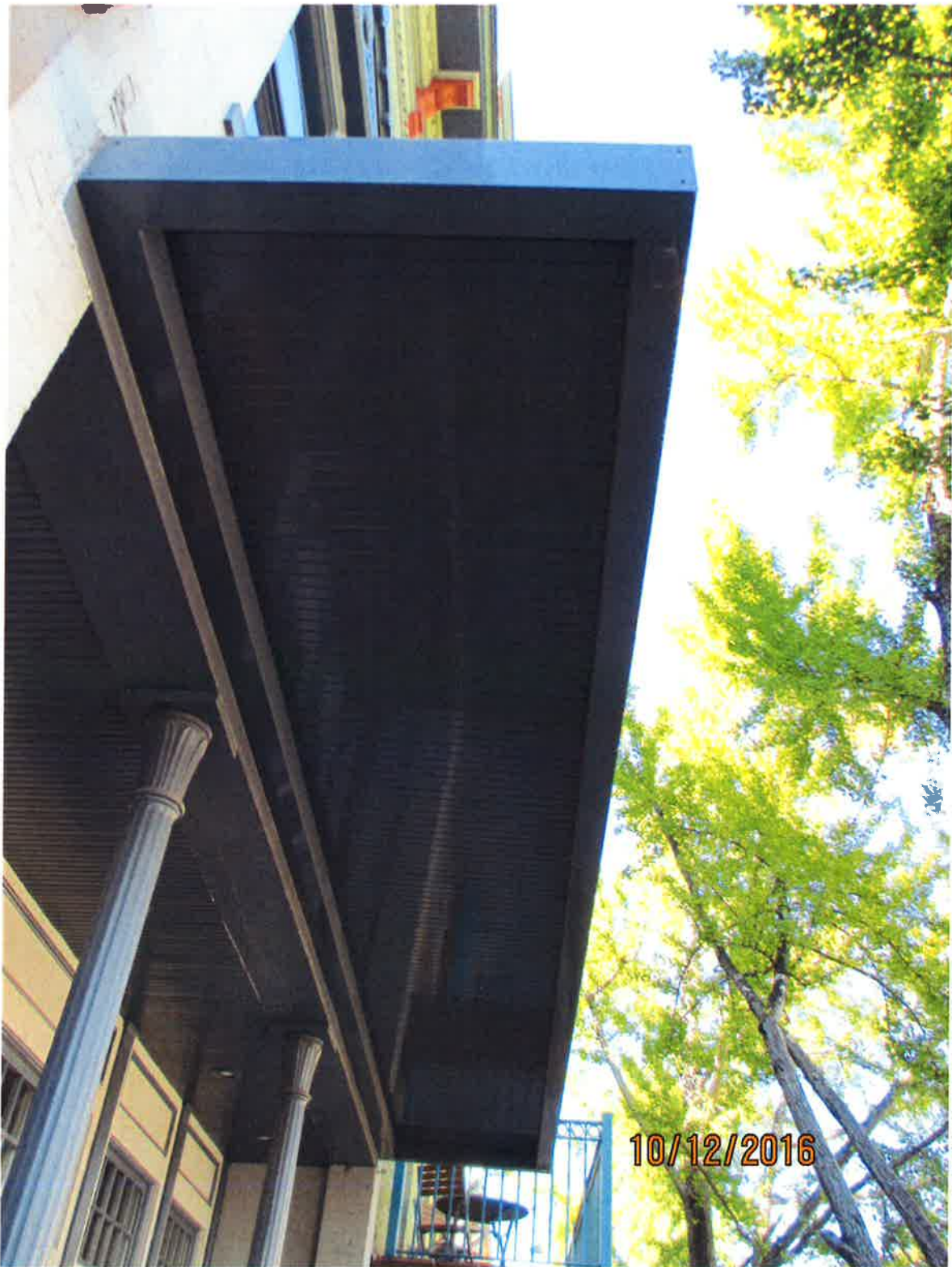
Metal "beadboard" installed at 24 S Perry Street
