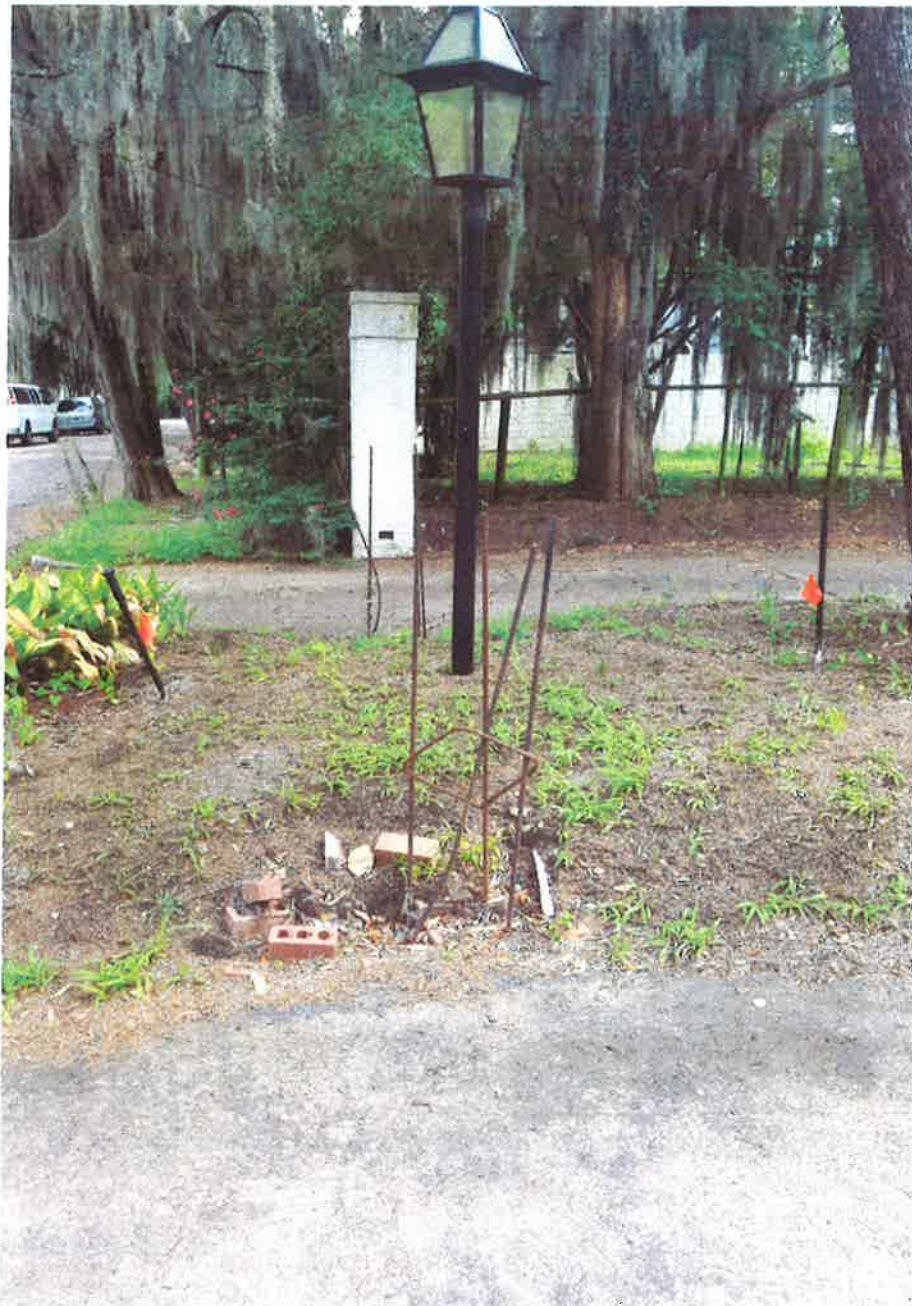
Current state of pillars
