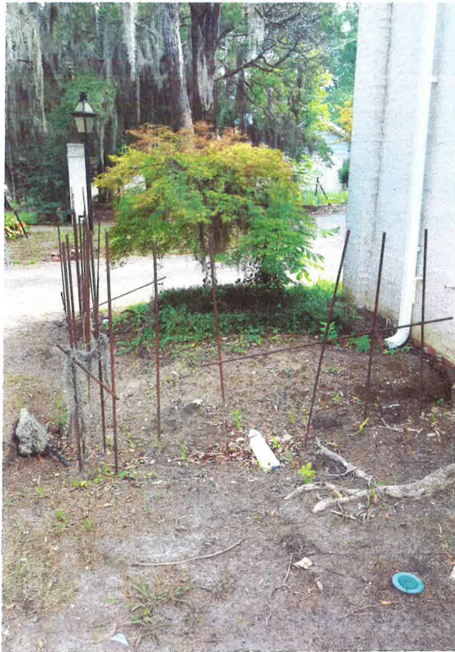
Current state of wall
