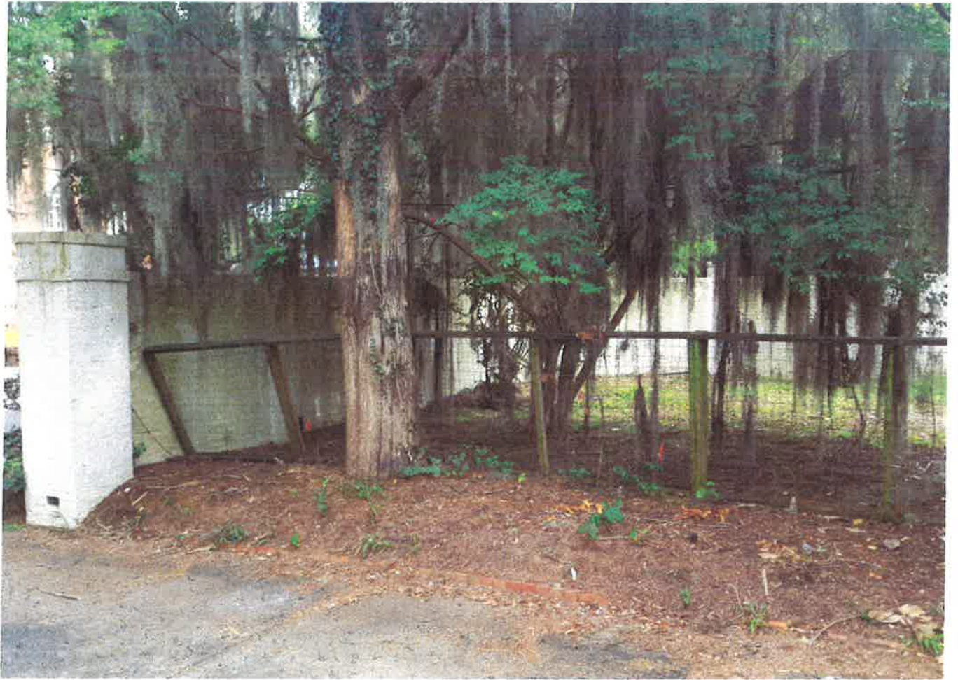
Existing wall on back and side of property
