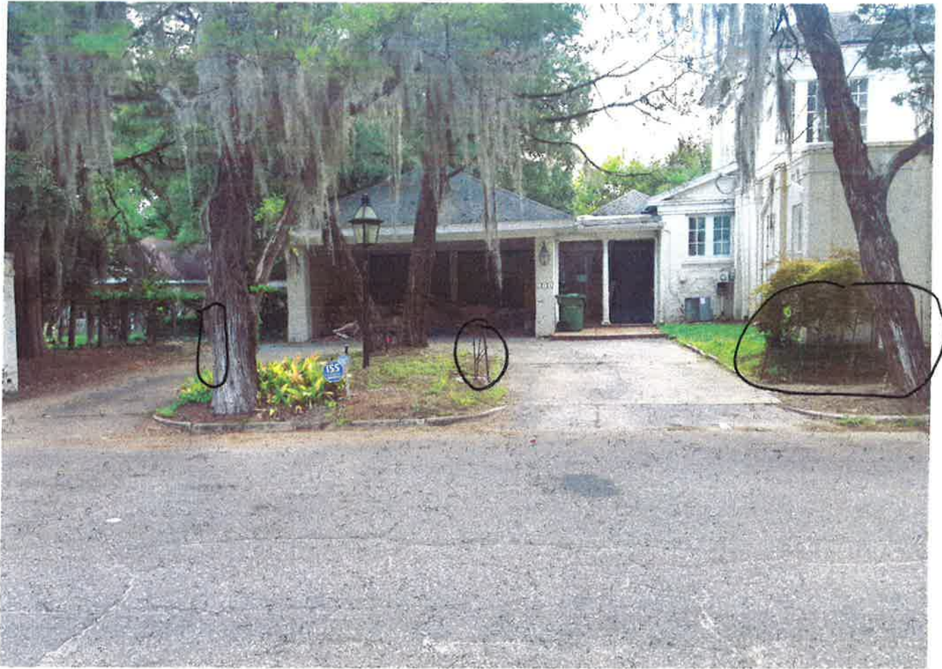
Current state of wall August 2016
