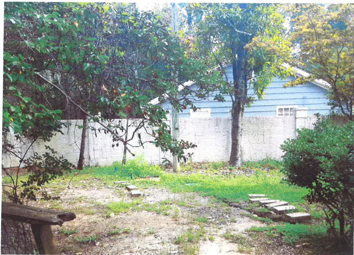
Existing wall on back of property
