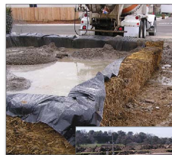
Figure 9. Hay bale and plastic washout pit
