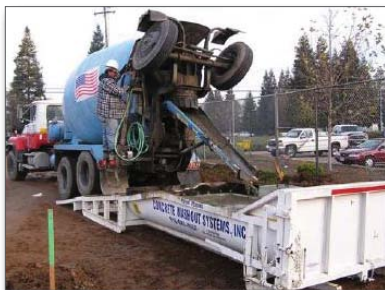
Figure 13. Mixer truck being washed out into a roll-off bin
