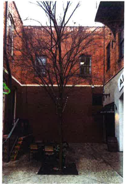
ALLEY EXISTING FACADE
