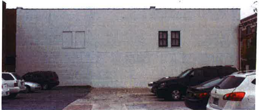
BIBB STREET EXISTING FACADE
