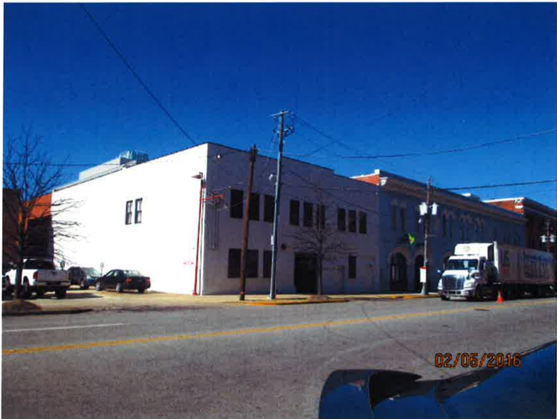
122 Commerce Street, Coosa and Bibb Street elevations
