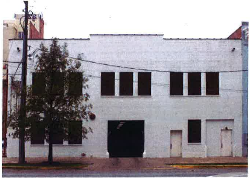
COOSA STREET EXISTING FACADE
