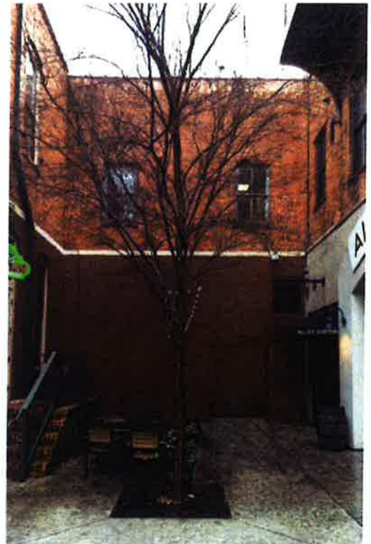
NEW WINDOWS, RE-USED FROM BIBB STREET FACADE
