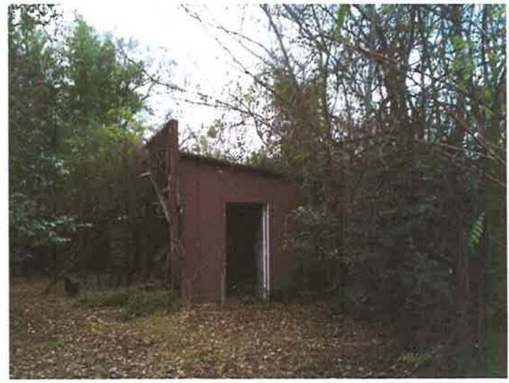
SHED IN BACK YARD
