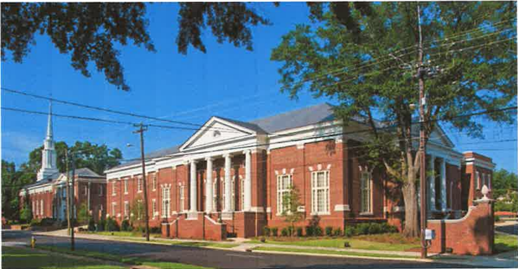
VIEW ALONG HULL STREET
