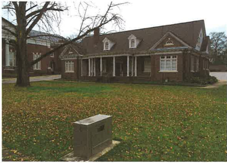
FRONT FAÇADE LOOKING SOUTH
