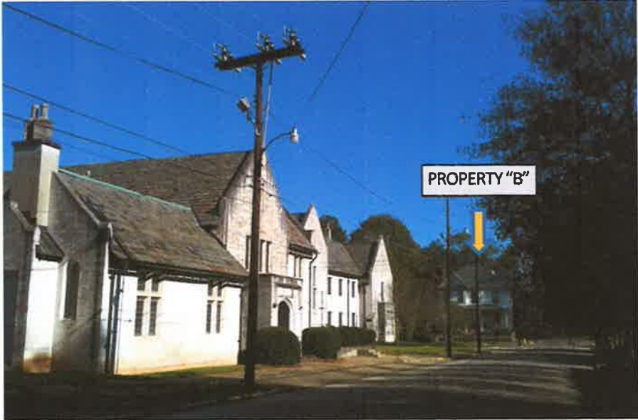
VIEW TOWARDS HULL ST. LOOKING DOWN CLANTON
