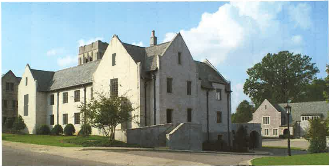
VIEW FROM CORNER OF PROPERTY @ HULL & CLANTON
