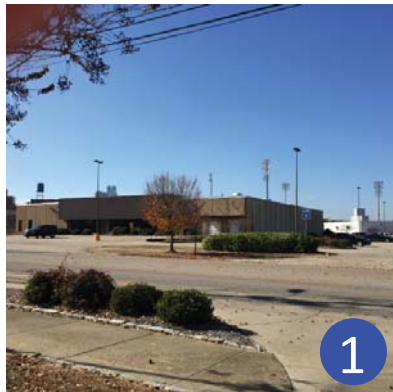
Vacant building on Block A, (30,000 s.f.)
