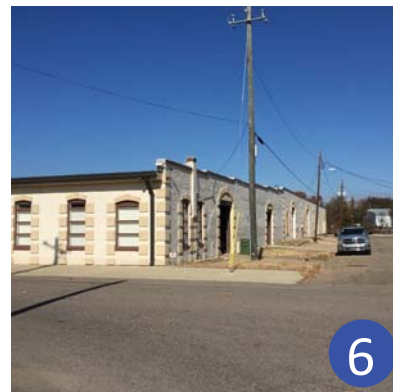
Single story warehouses north of site. N. Lawrence Street at Randolph, northwest corner
