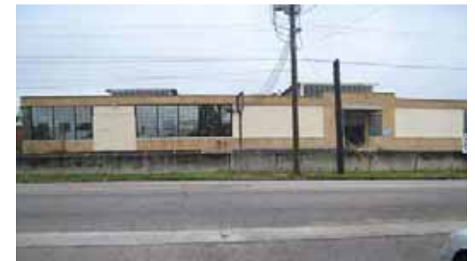
Vacant National Linen Service building
