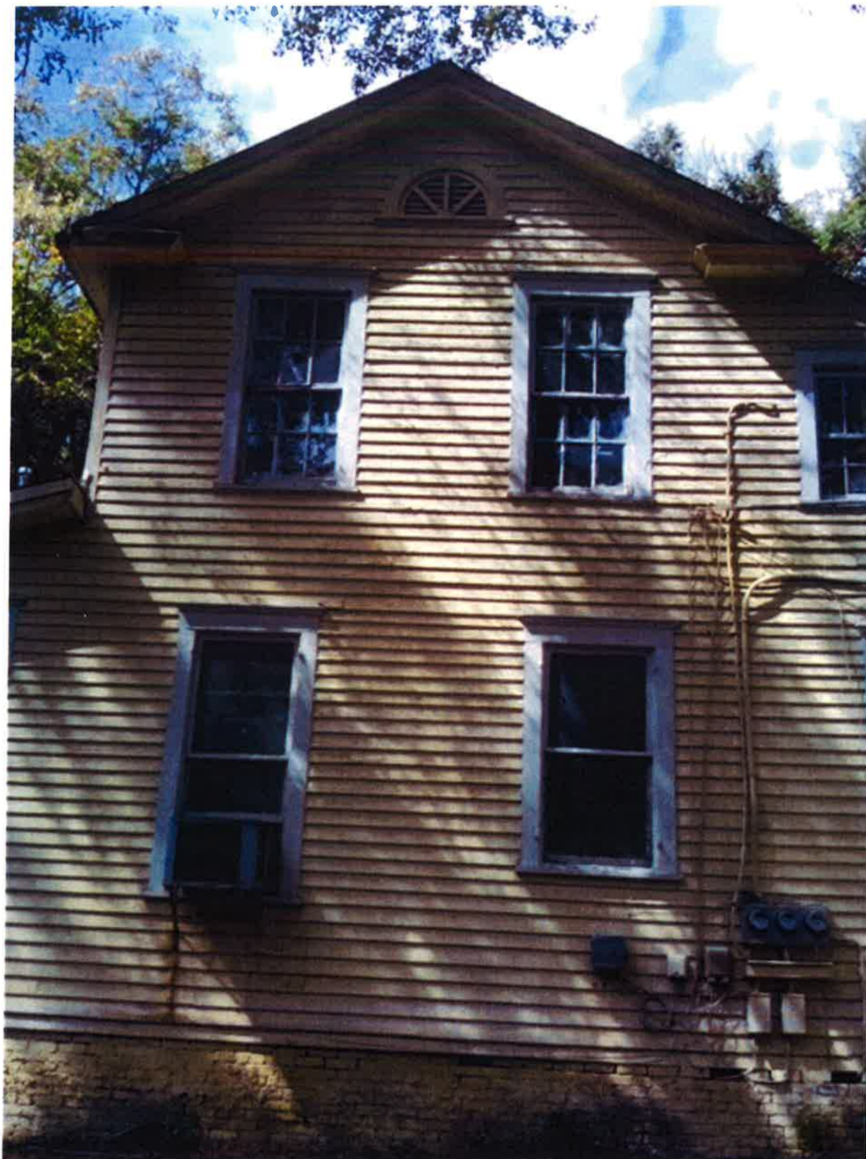
Left side (notice louver to be matched on addition)
