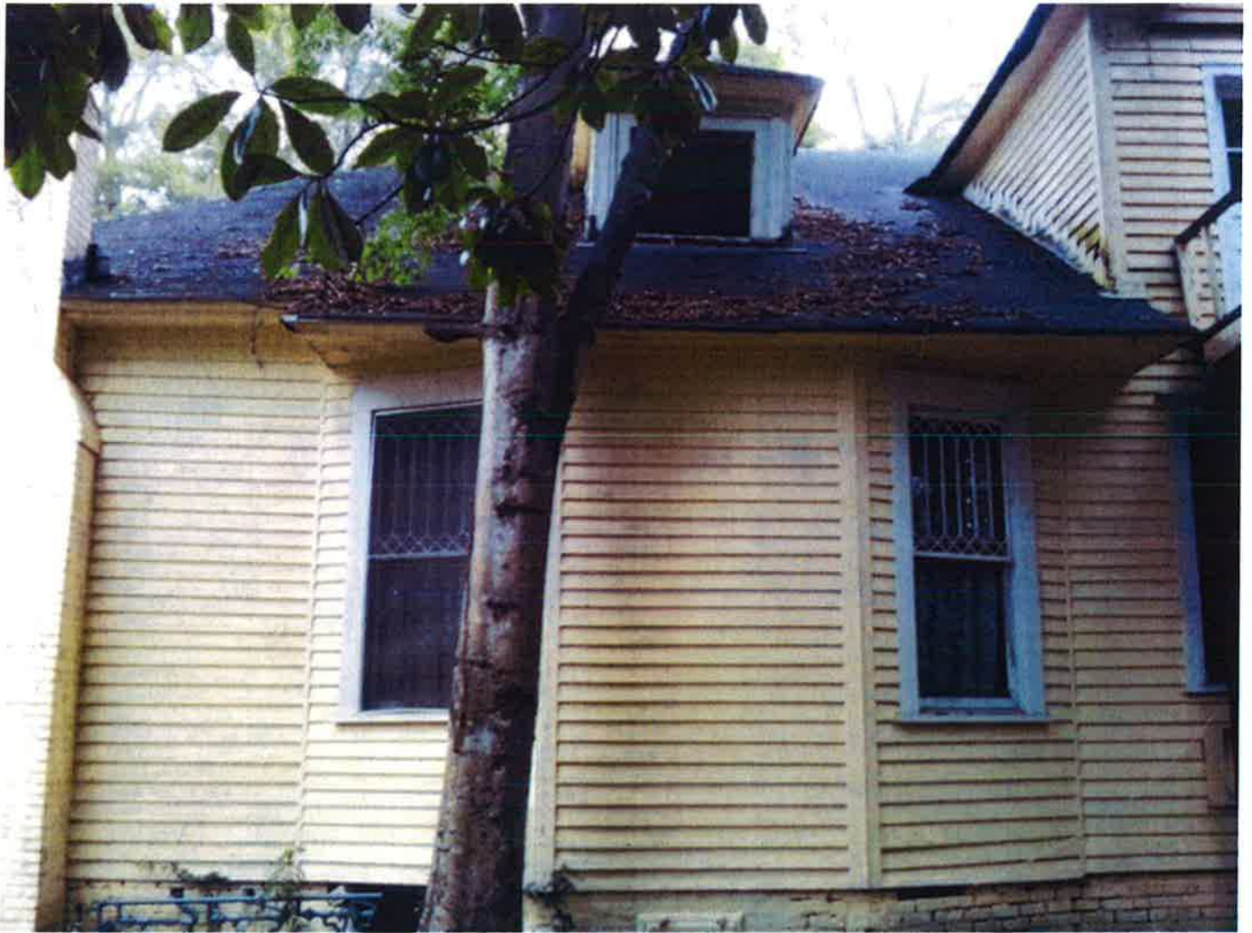
Right side showing dormer above dining area
