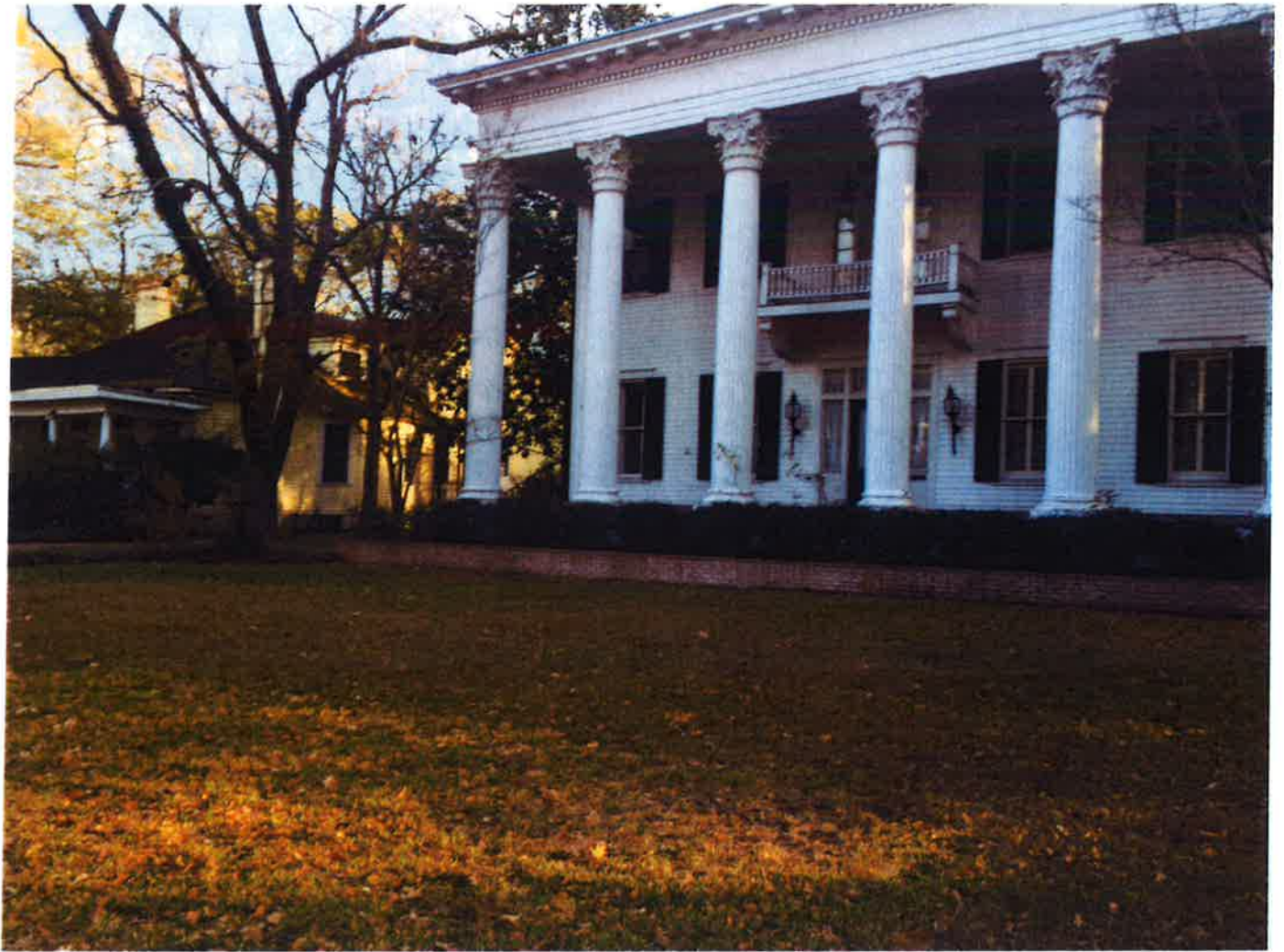
Home to Right of 740 Felder Avenue
