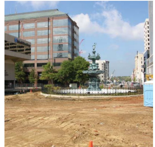
Construction on the redesigned Court Square began in September 2006
