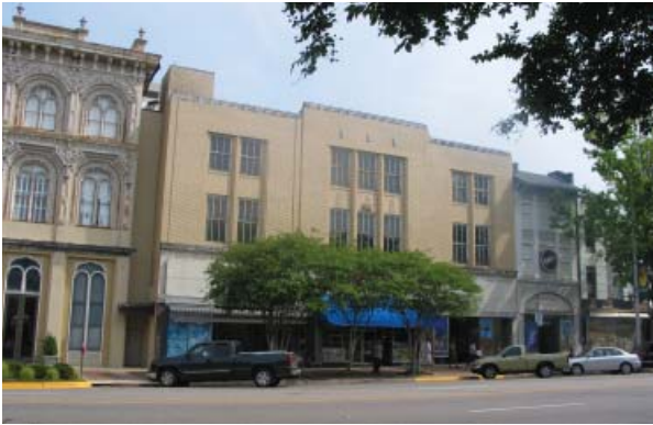
Dexter Avenue, existing conditions
