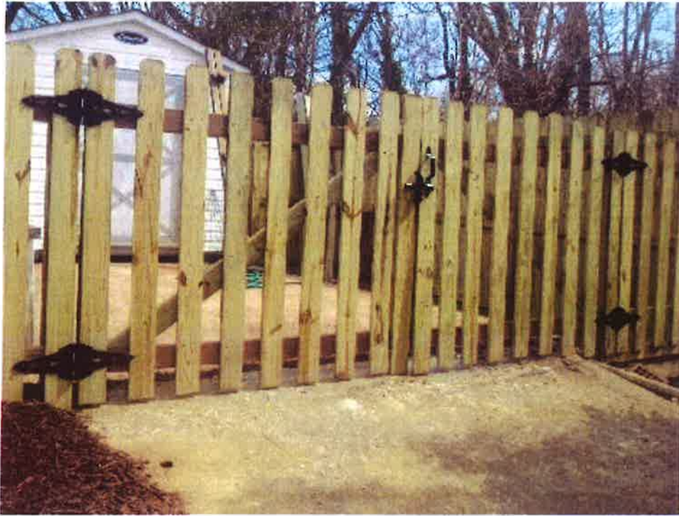
G. Example of unpainted 4' 4" Cyprus fencing material
