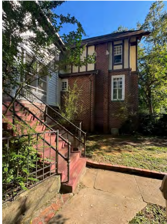
Figure 3d: Existing conditions of the project area (West elevation) at 831 Felder Ave.
