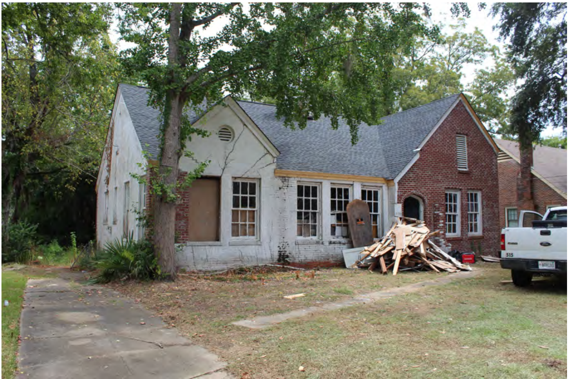
Figure 1b: Existing windows at West façade of 3135 Lexington Rd., 09/26/2024
