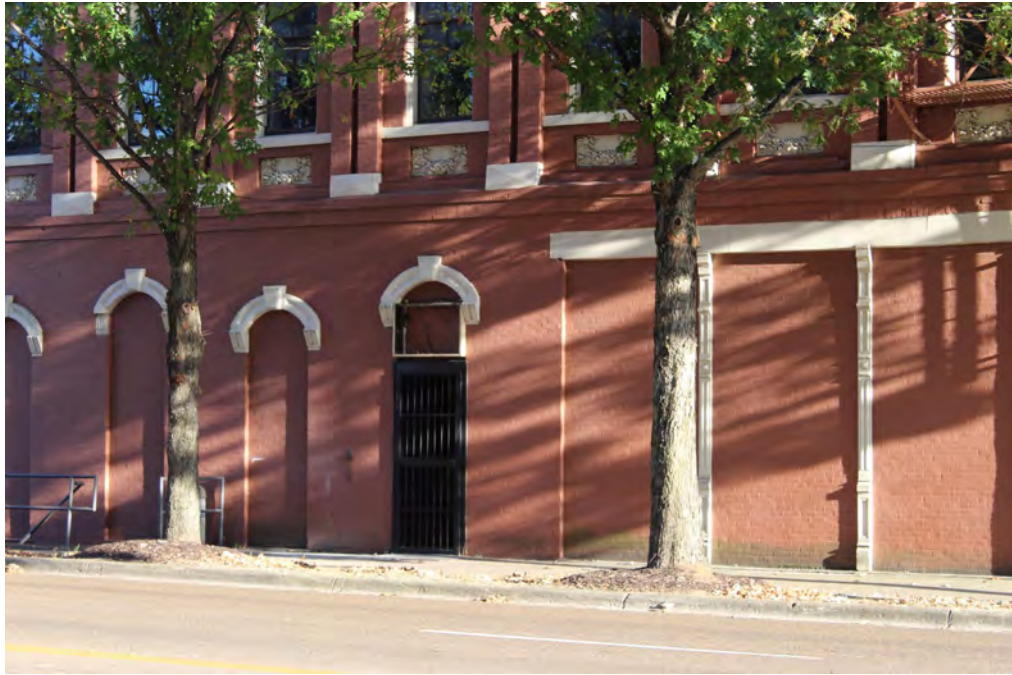
Figure 4d: Project area at northwest elevation, 82 Commerce St., 10/24/2024
