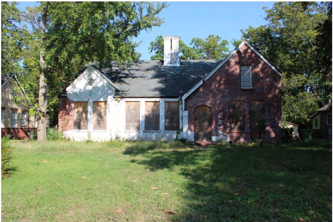
Figure 1a: 3135 Lexington Ave, West façade, 09/18/2023
