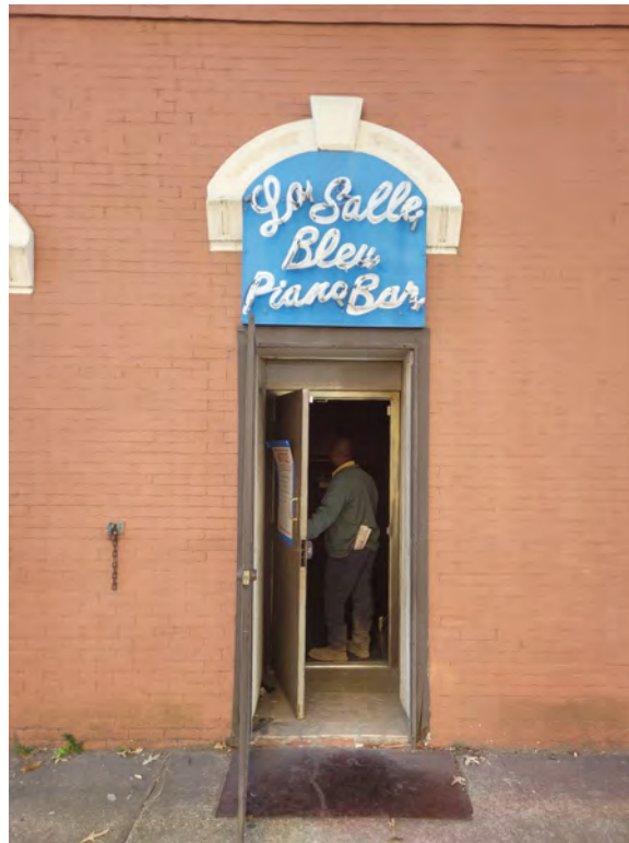
Figure 4c: Project area at northwest elevation, 82 Commerce St., 10/24/2024
