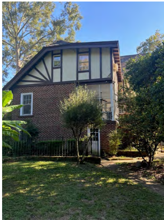
Figure 3e: Existing conditions of the project area (North elevation) at 831 Felder Ave.
