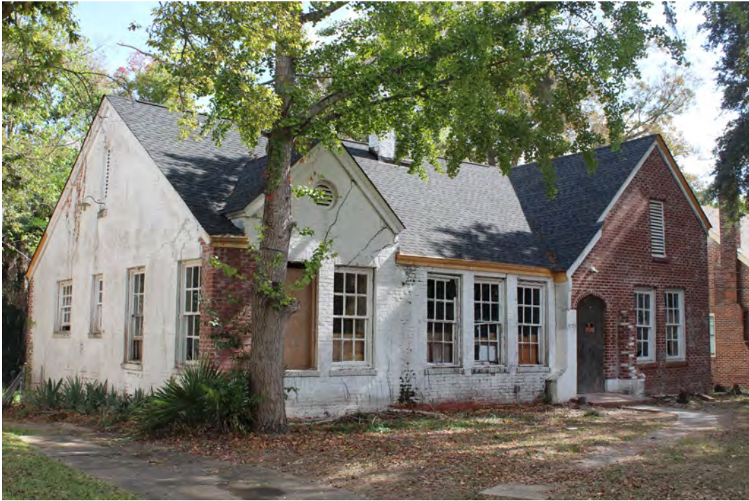
Figure 1g: Location of proposed new window (top left) on the North elevation
