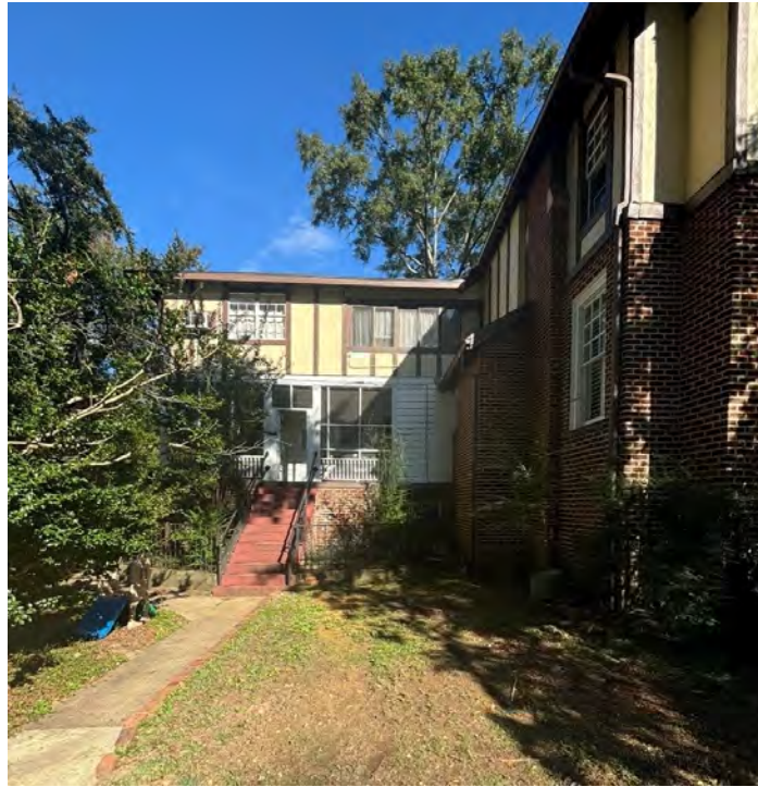
Figure 3b: Existing conditions of the project area (rear inside corner of the home) at 831 Felder Ave.
