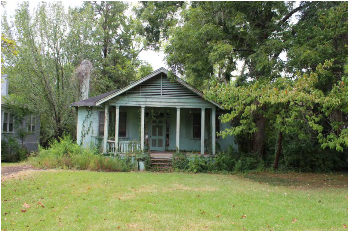
Figure 2a: 620 Ponce de Leon Ave, North façade, 09/05/2024
