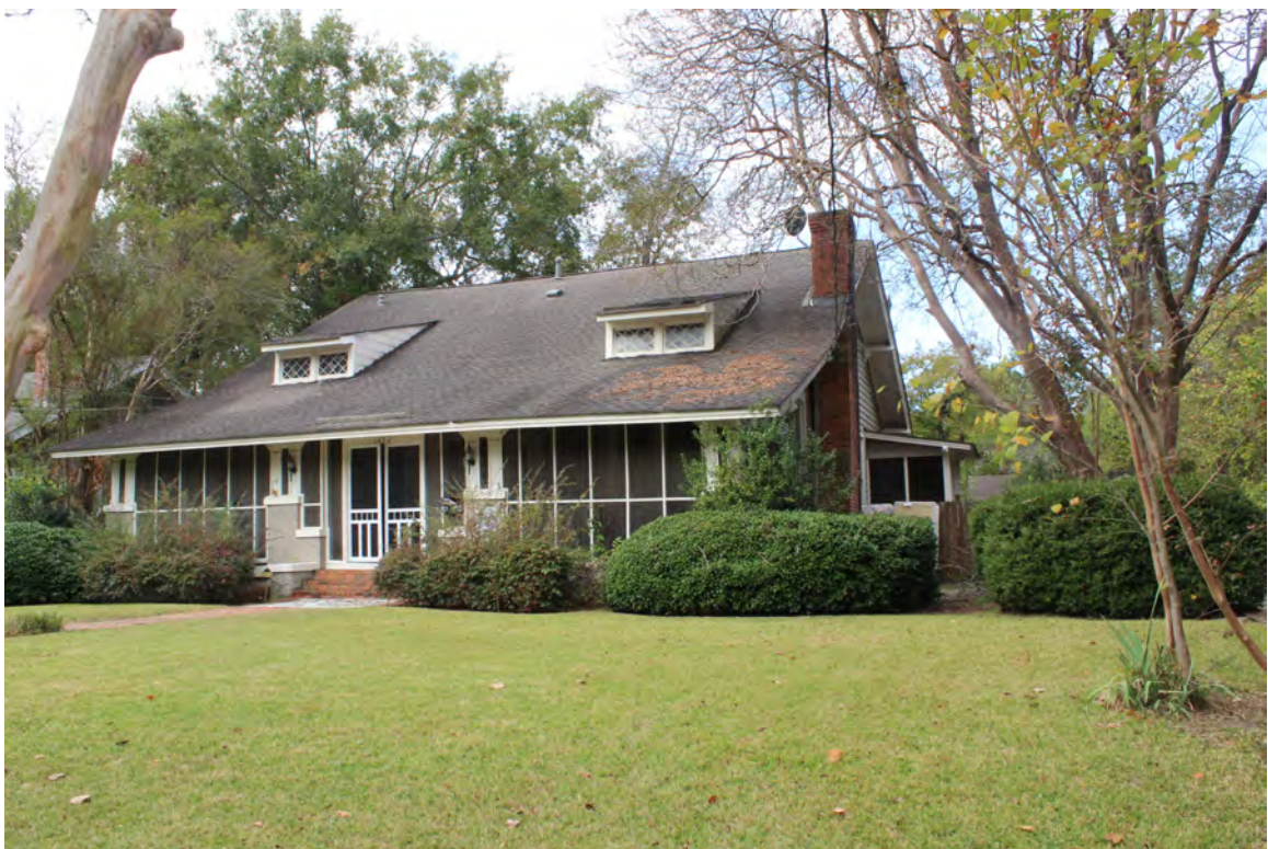
Figure 5b: East façade and north elevation with chimney in context, 10/31/2024
