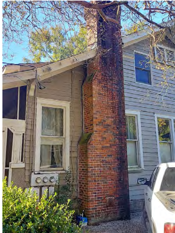
Figure 5c: Chimney in context, 1852 Graham St., 10/22/2024
