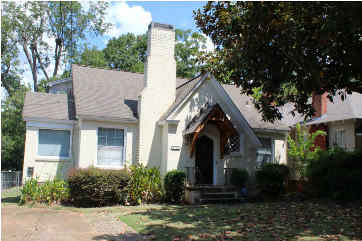
Figure 6a: West façade of 2119 St. Charles Avenue, 09/03/2024
