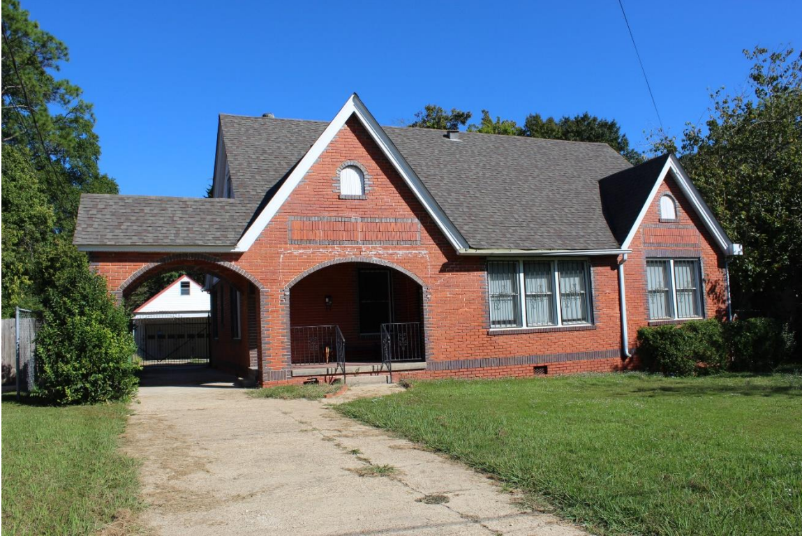
Figure 40: West façade with view of garage in rear.
