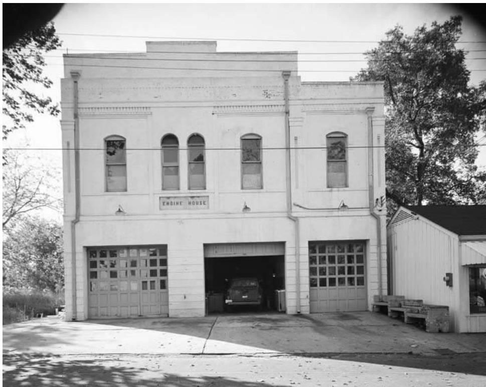
Figure 10: N. Façade of Scott Street Firehouse, 10/25/1967, by John E. Scott. Note alterations to the doors at ground level and roof.
