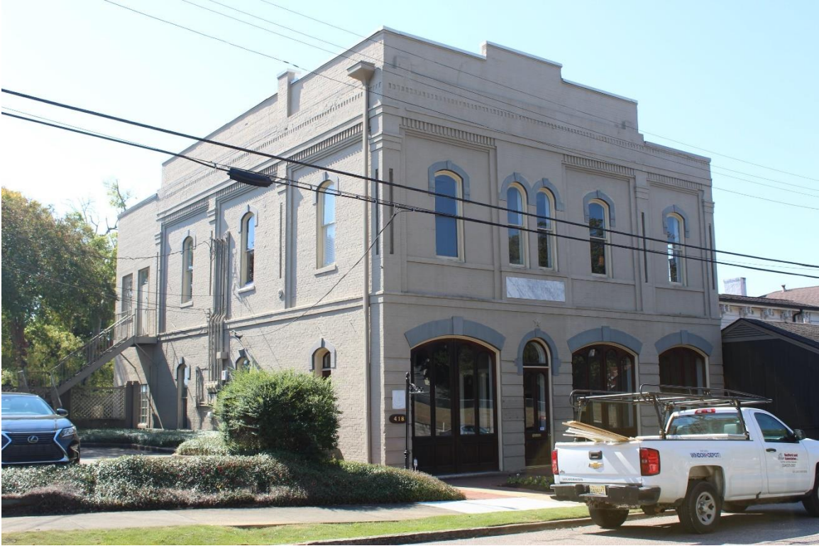
Figure 13: N. Façade and east elevation of Scott St. Firehouse at 418 Scott Street, 10/25/2024.
