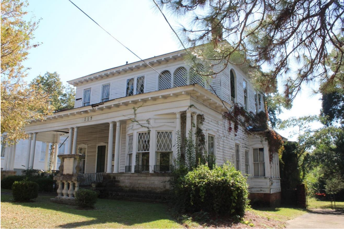
Figure 21: N. façade and west elevation of the Crommelin Jackson House at 119 Fred Gray Avenue, 10/25/2024.
