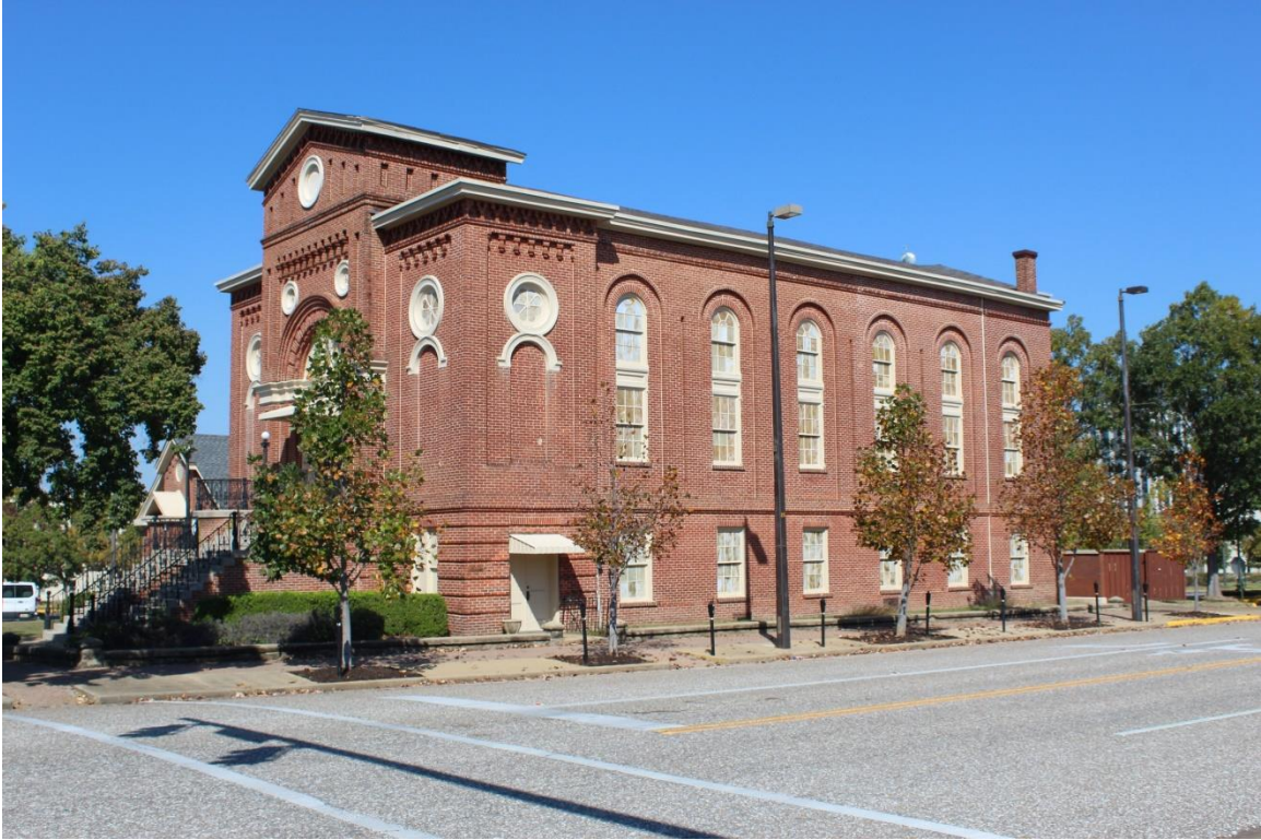
Figure 15: Southeast elevation of Kahl Montgomery Synagogue, now Catoma St. Church of Christ, 10/25/2024.
