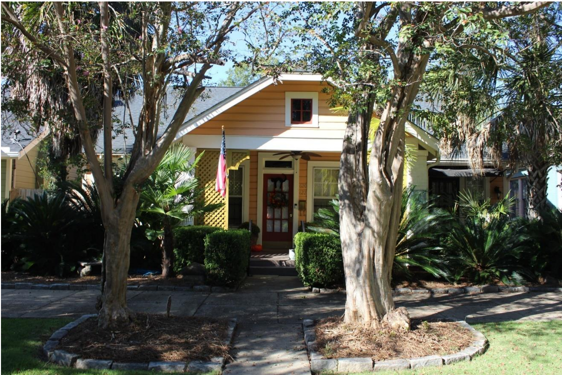
Figure 38: Main entry detail, 10/10/2024.
