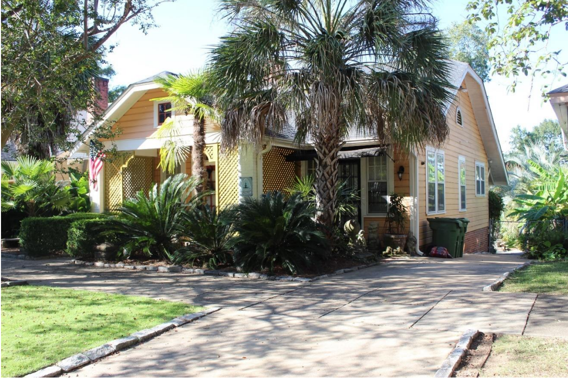
Figure 35: South facade and east elevation, 10/10/2024.
