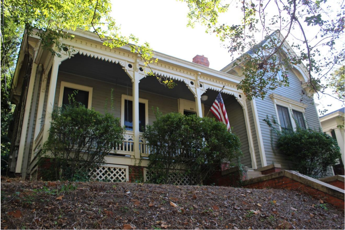
Figure 34: Decorative porch details, 10/10/2024.
