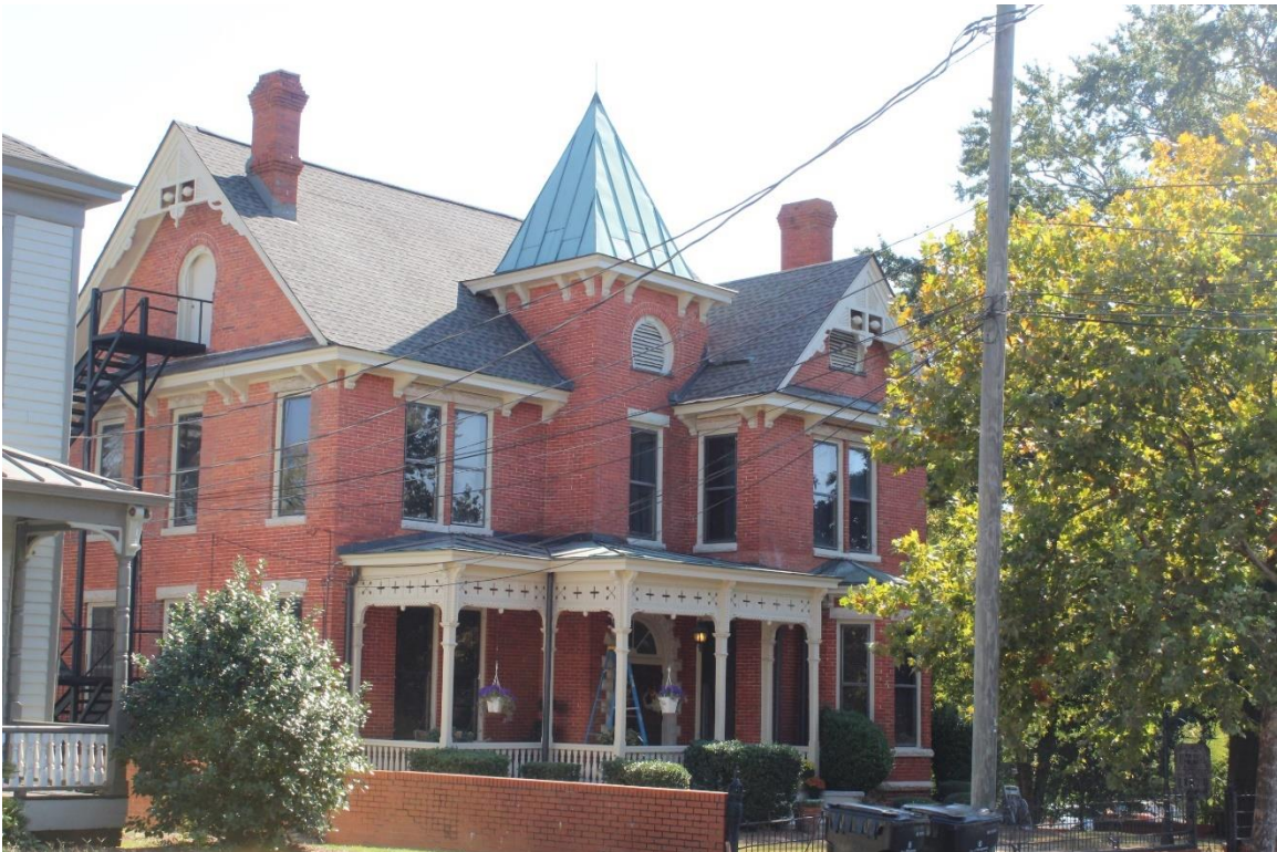
Figure 30: West façade of the Stay House at 631 S. Hull St., 10/25/2024.
