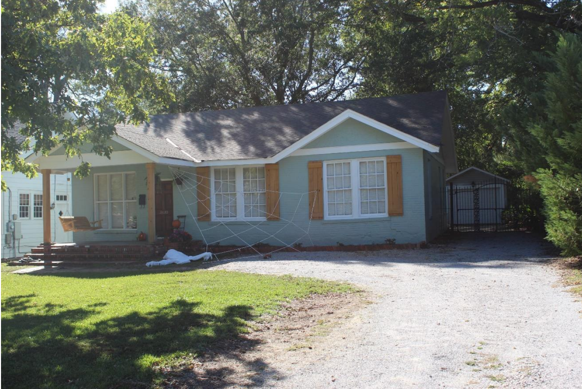
Figure 39: East façade of 3130 Montezuma Rd., 10/10/2024.
