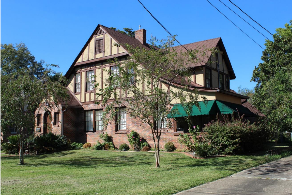
Figure 43: South facade and east elevation.
