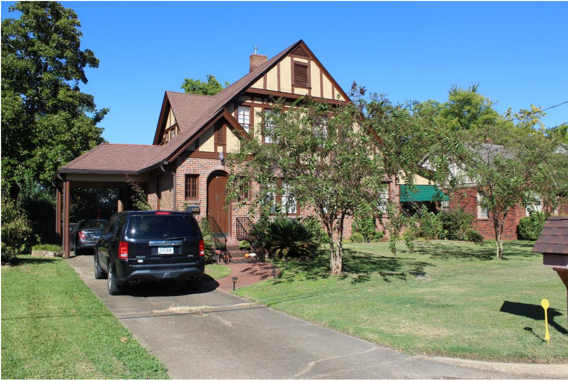
Figure 44: South facade and west elevation.
