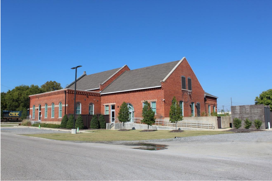
Figure 7: South and East elevations (rear) of Legacy Hall, 10/25/2024.
