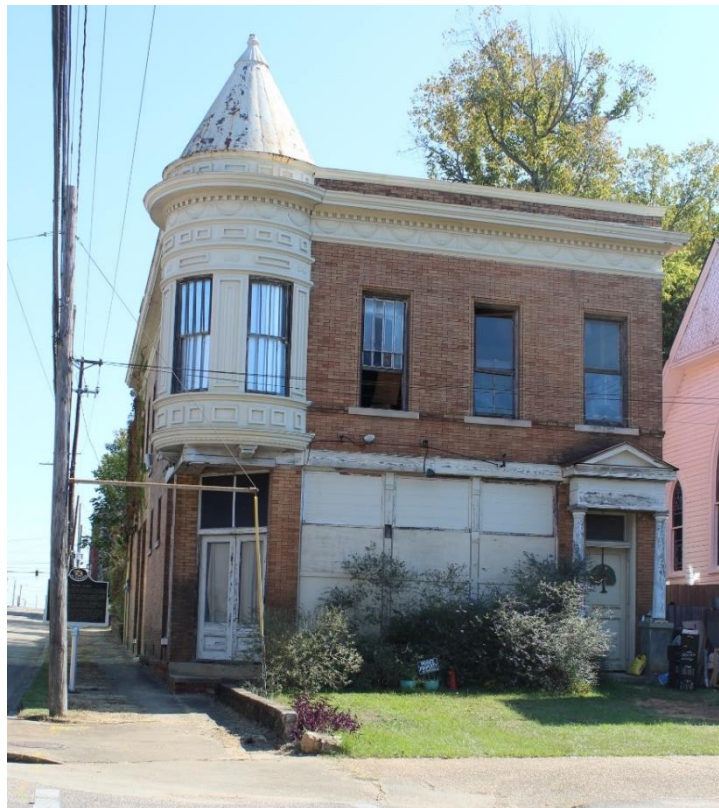
Figure 24: West façade of the Tulane Building at 800 High St., 10/25/2024.
