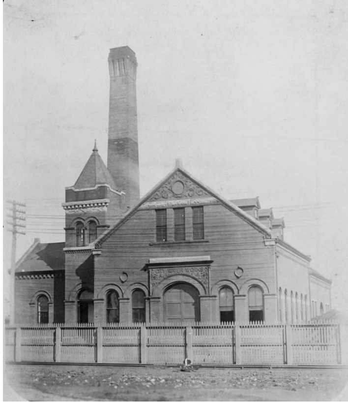
Figure 5: North Court Water pumping station at 608 N. Court St., c. 1900. Photographer: John E. Scott. Courtesy of Alabama Dept. of Archives & History: https://digital.archives.alabama.gov/digital/collection/photo/id/31436/ .
