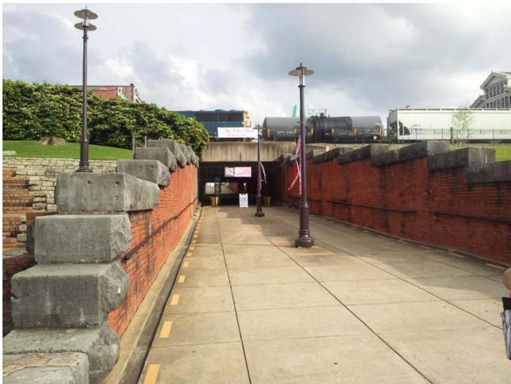
Figure 4: Looking back through the tunnel up toward Commerce Street.
