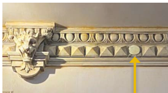
Figure 2: Sprinkler heads and other equipment can be selected and placed to have minimal visual intrusion with no impact on functionality, such as these fixed (left) or concealed (right, with arrow) sprinkler heads. Photos: Marilyn Kaplan
