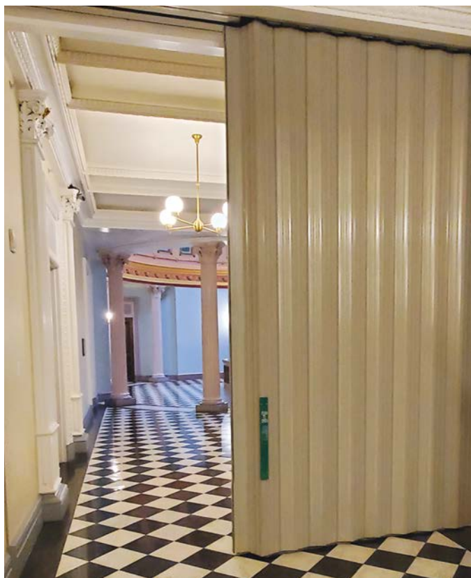
Figure 4: Creative life- and fire-safety code solutions may be required for special buildings and conditions, such as the use of an automatic accordion type, horizontal-sliding fire and security door to meet code requirements. Concealed when not in use, such systems can provide up to a 3-hour fire-resistance rating. Photo: U.S. General Services Administration
