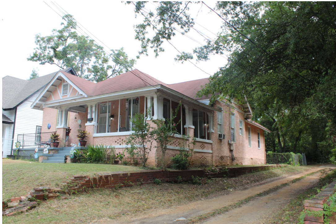
Figure 2a: West façade, 1223 S. Hull Street, 09/05/2024 (note the alley at right)
