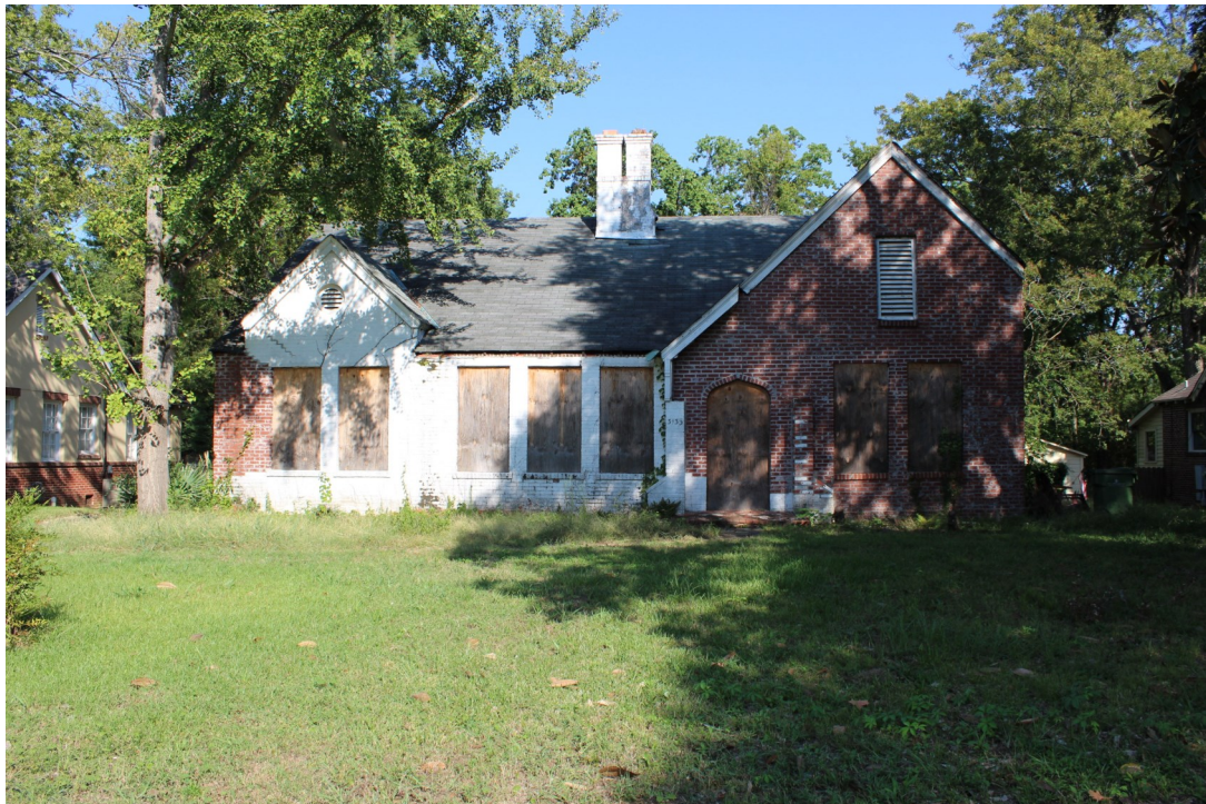
Figure 3a: 3135 Lexington Ave, West façade, 09/18/2023
