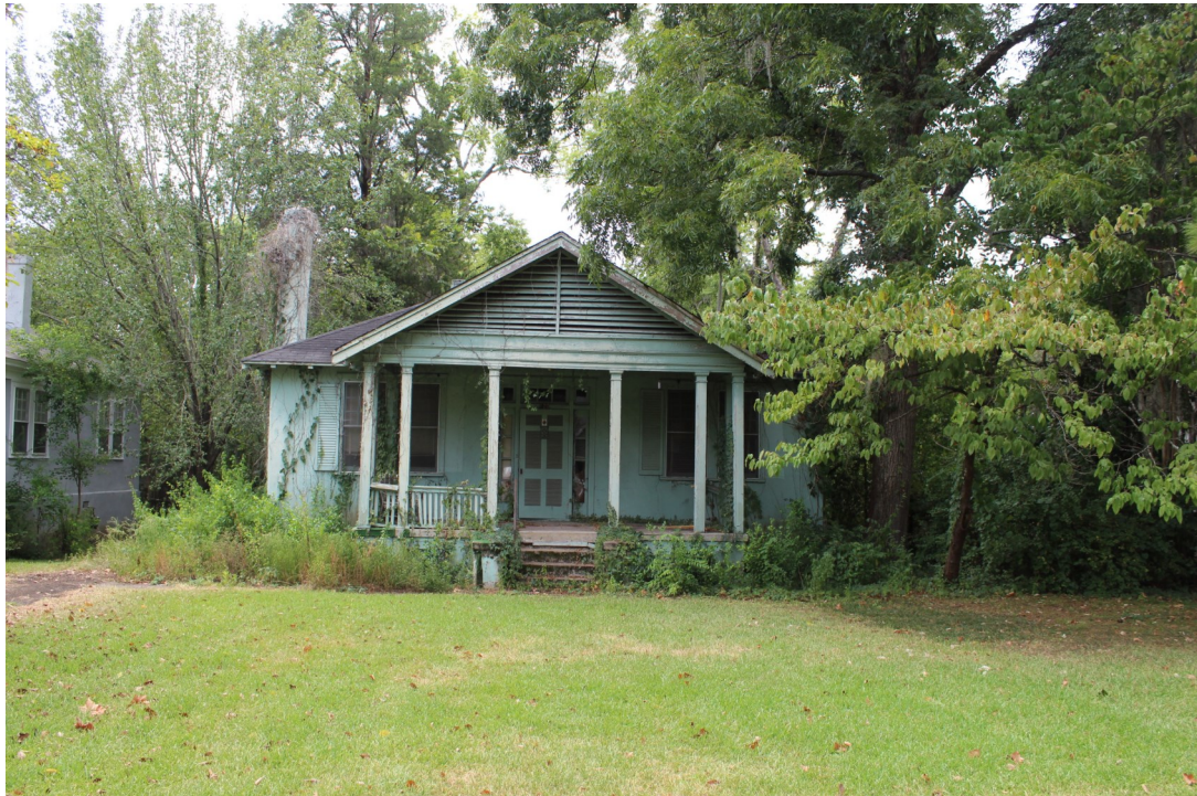
Figure 4a: 620 Ponce de Leon Ave, North façade, 09/05/2024
