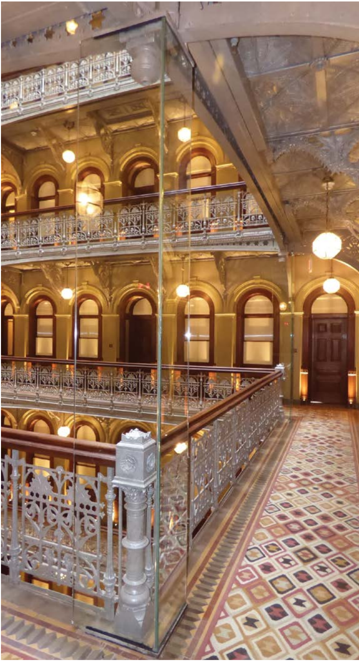
Figure 21. The photograph on the right illustrates partial deployment of vertical fire curtains activated as part of a fire alarm and detection system. In this installation, a combination of fixed glazing and smoke curtains to separate the open corridors from the multi-story atrium permitted the stunning historic atrium space to remain largely unaltered and the corridors to be included in the building's egress calculations in meeting code requirements. Photo: Higgins Quasebarth & Partners, LLC
