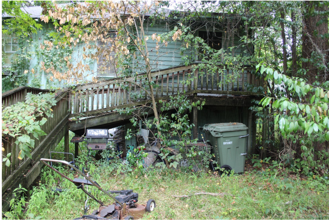
Figure 4d: 620 Ponce de Leon, existing rear deck and ramp
