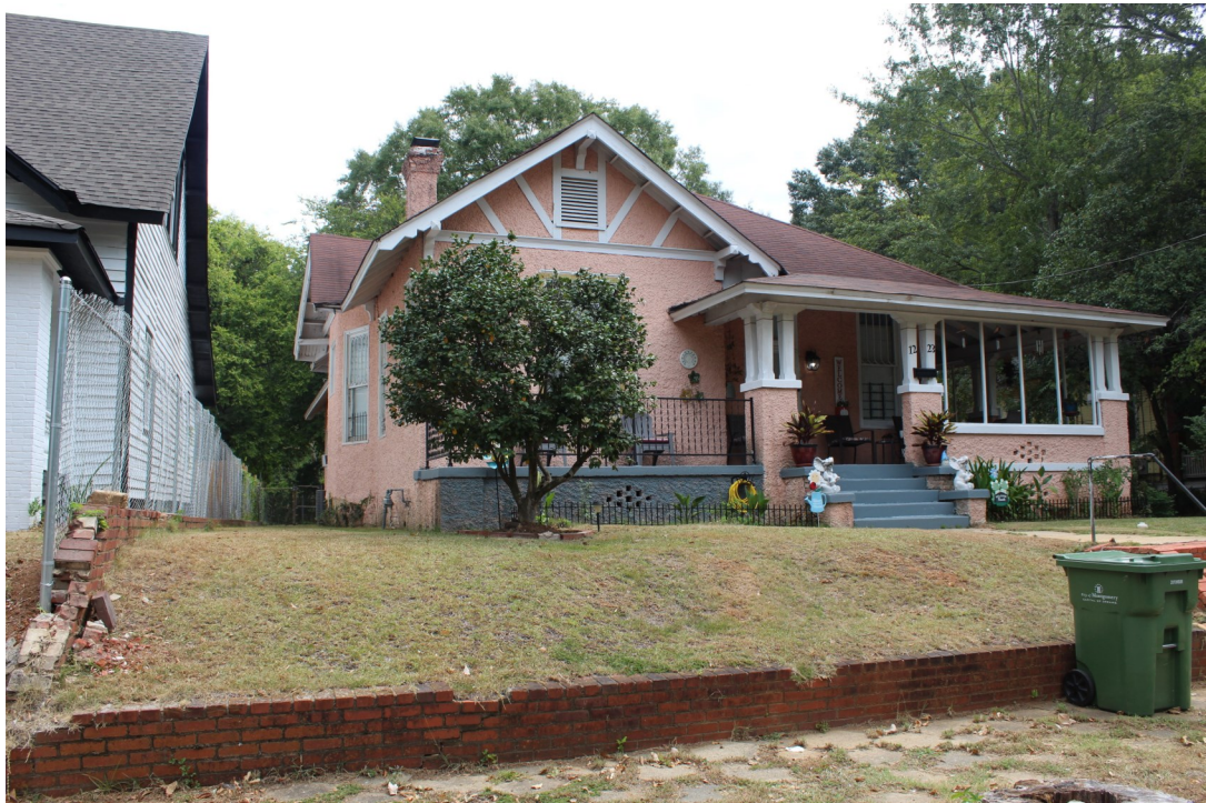
Figure 2b: West façade with fence section at left, 1223 S. Hull St., 09/05/24
