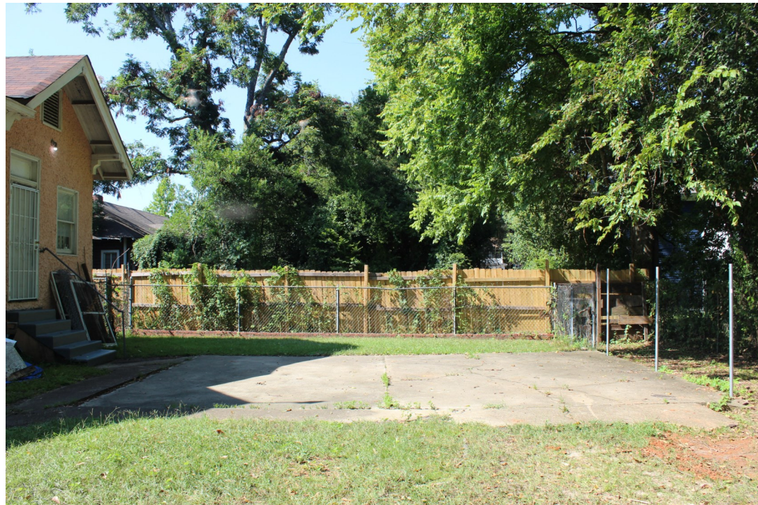
Figure 2e: Rear portion of fence, 1223 S. Hull St., 09/05/24
