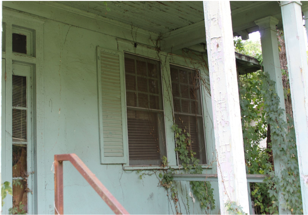
Figure 4b: 620 Ponce de Leon Ave, typical window (in fair condition)
