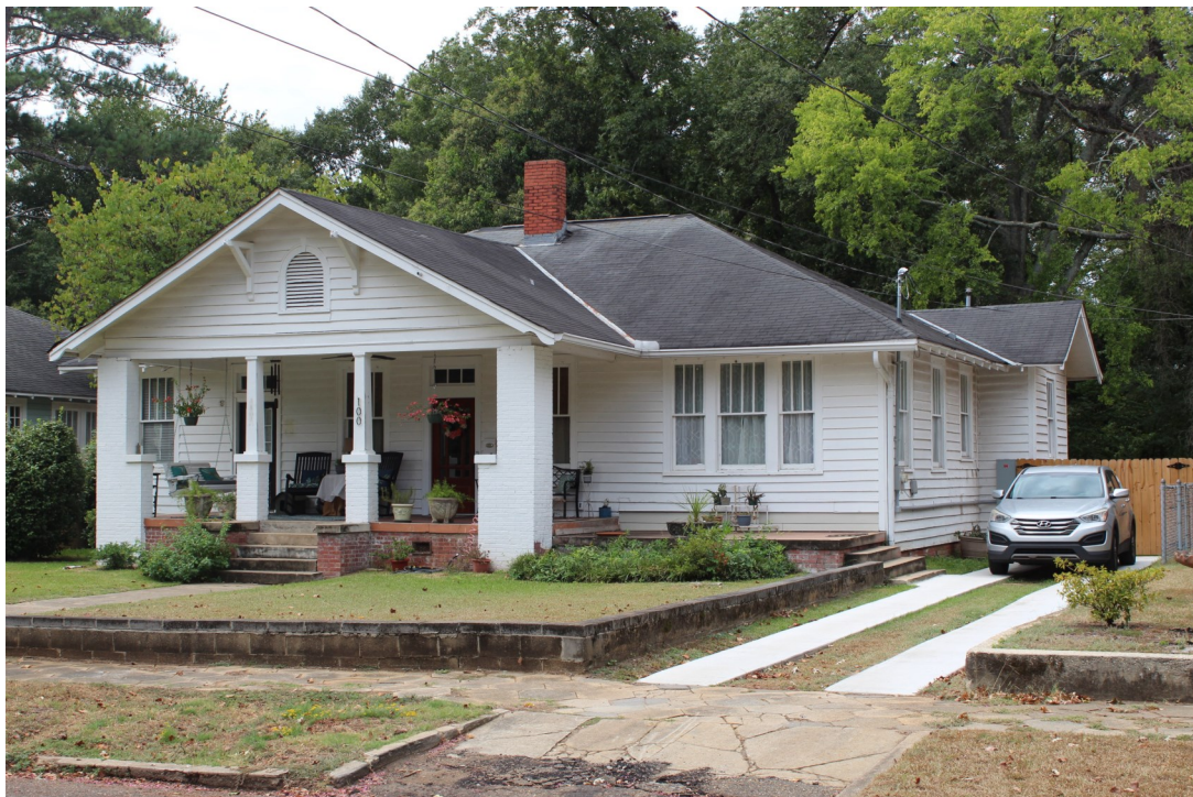
Figure 1a: East façade, 100 S. Capitol Pkwy, 09/05/2024
