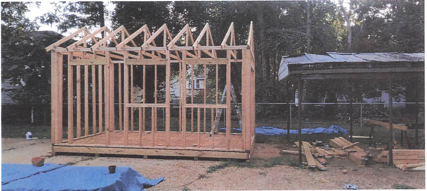
2219 St. Charles Ave. (Capitol Heights), outbuilding in progress in rear yard, 07/03/2024
