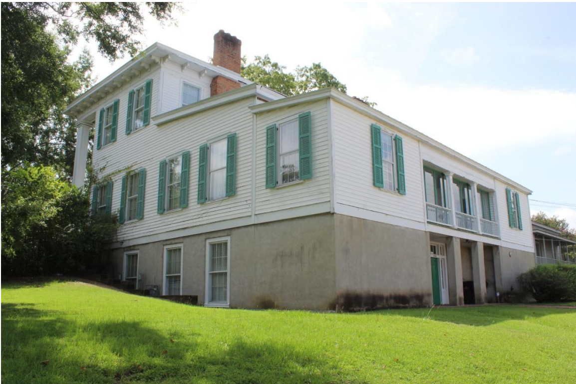
Figure 9: Rear of c. 1850s Molton House.
