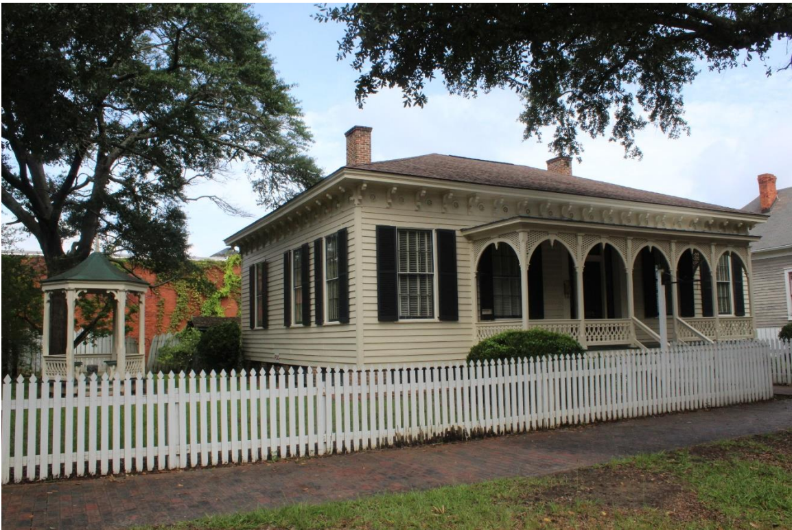
Figure 3: DeWolfe Cooper cottage, c. 1850s, at 309 N. Hull Street.
