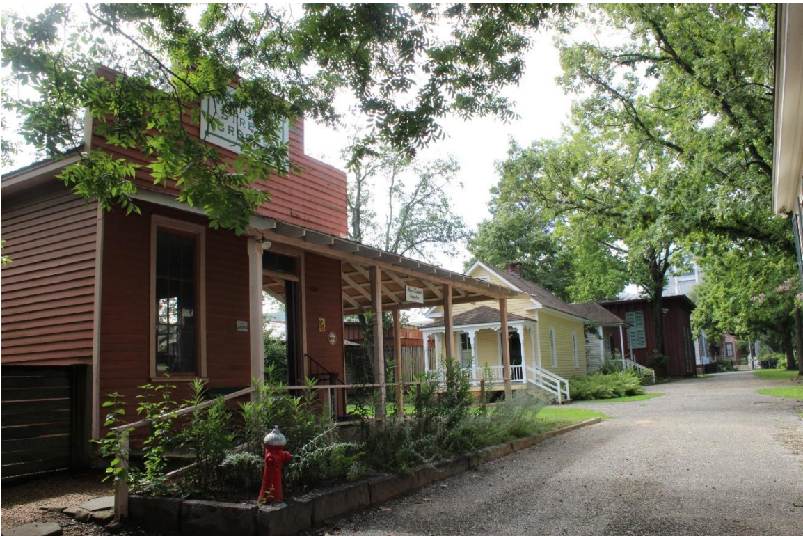
Figure 5: A segment of the "Living Block." Rural grocery store, c. 1892, in foreground; yellow 1880s shotgun house beyond.
