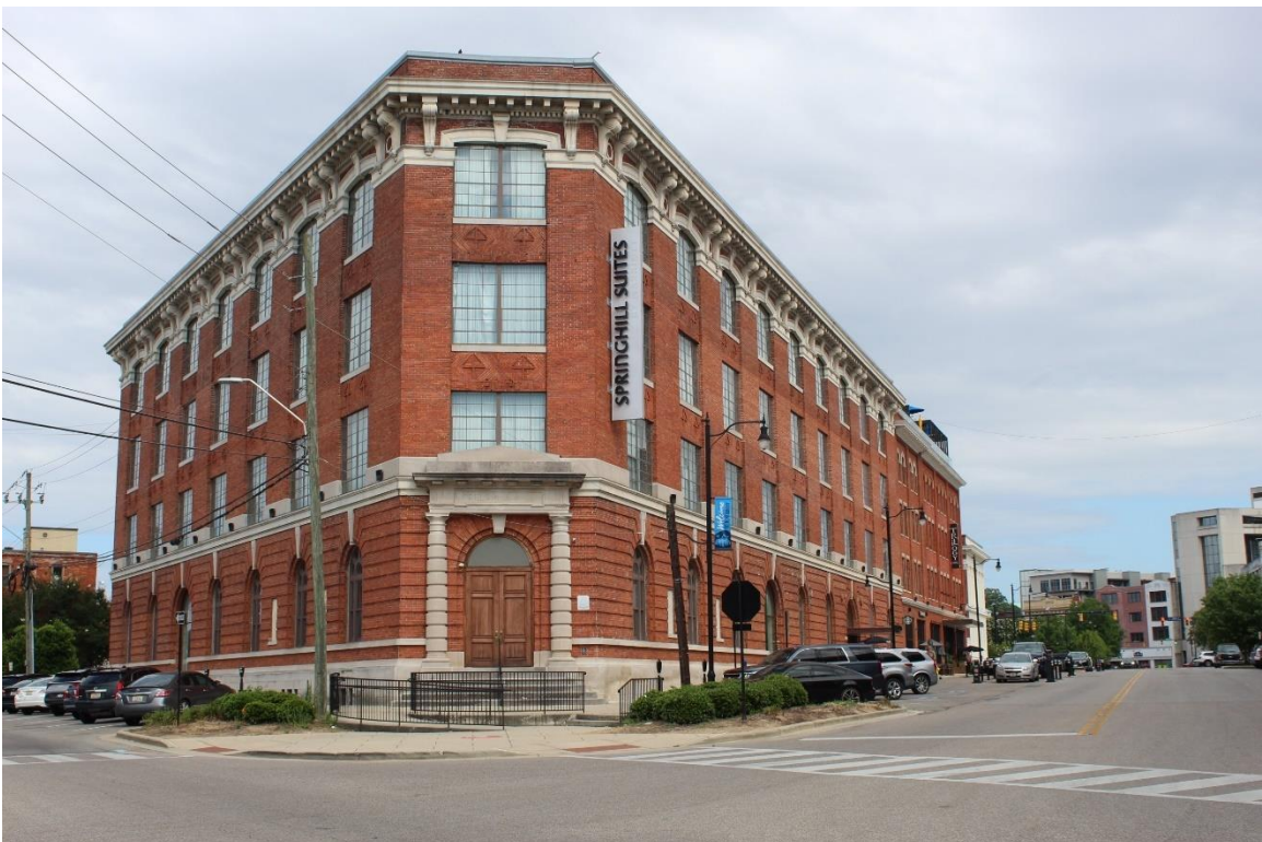
Figure 20: Northwest corner of Former Schloss & Kahn building, constructed 1907, at 152 Coosa St.
