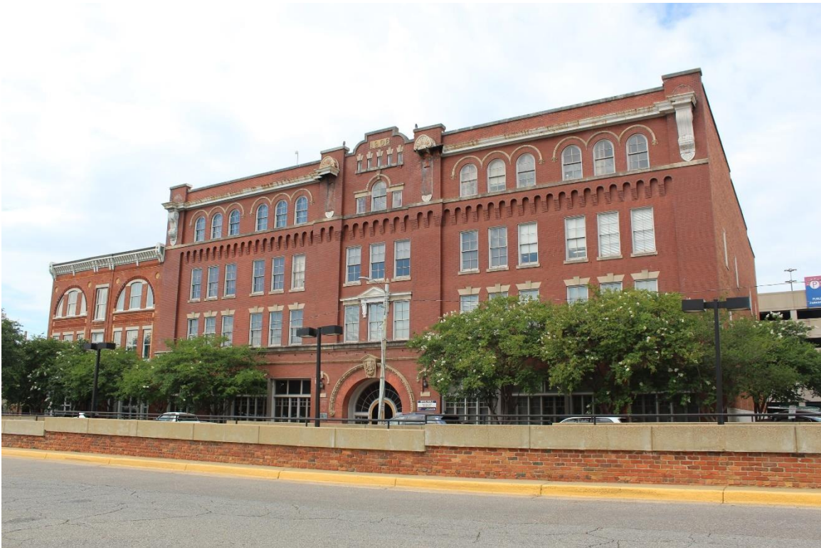
Figure 6: 4-story Hobbie Building, constructed c. 1903-1906.
