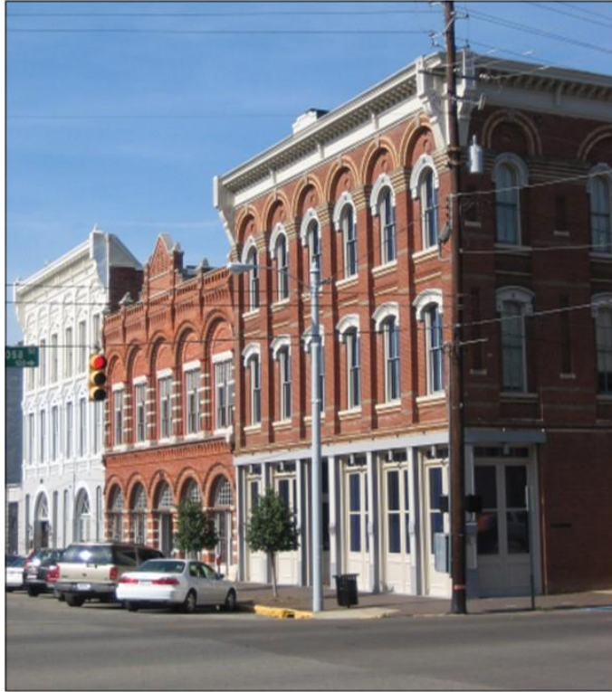
Figure 9: From right to left—McIntyre Building at 200 Commerce St., built c. 1890; old Implement Store at 210 Commerce St., built 1894-95; and the Durr-Fillauer-Schloss & Kahn Building, built c. 1890-1900.
