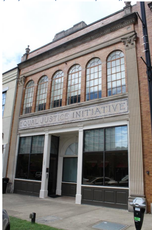
Figure 12: Whitfield-Massey Draughon Building (Now Equal Justice Initiative HQ), constructed in 1928.
