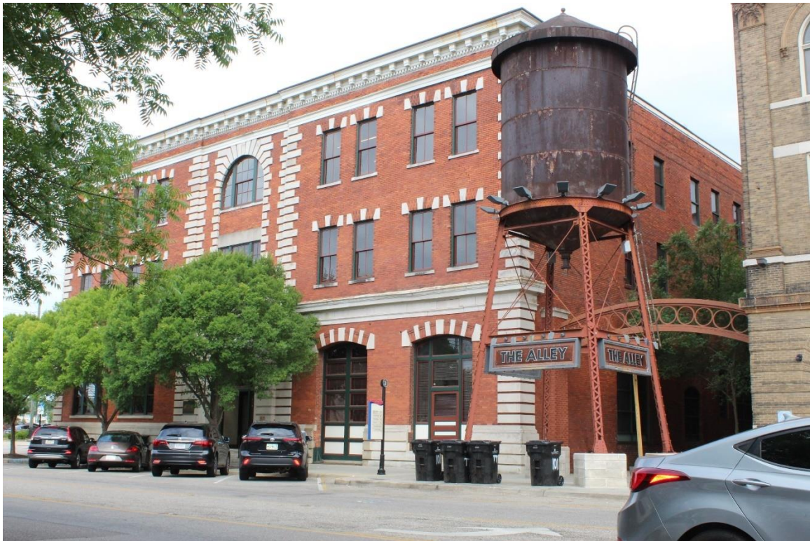
Figure 18: North elevation of Former Winter-Loeb Grocery Co. at 105 Tallapoosa St., built in 1895.
