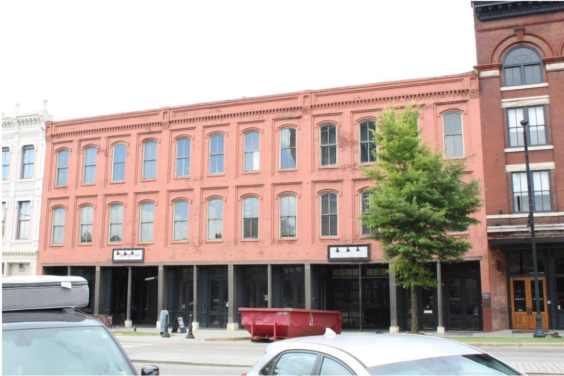
Figure 15: Old Mercantile Business Products building.
