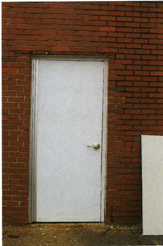
121 N. Goldthwaite Street (Cottage Hill), egress doors on north elevation, 06/05/2024
