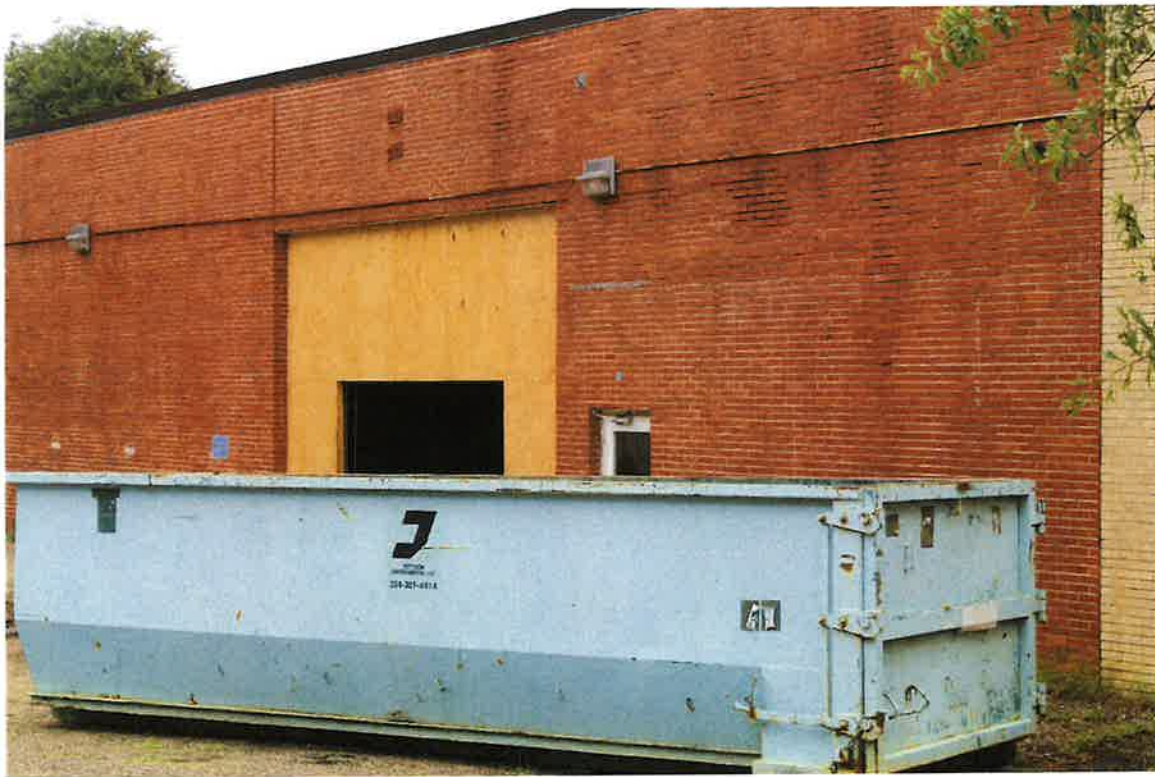
121 N. Goldthwaite Street (Cottage Hill), garage and egress doors on north elevation; boarded garage door opening on south elevation, 06/05/2024
