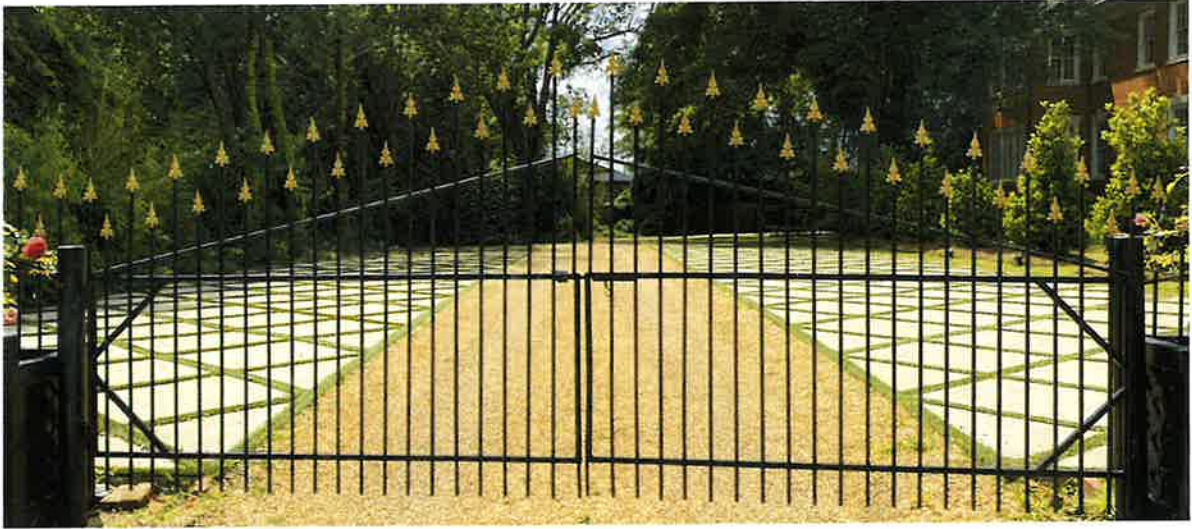
Existing Front Gate
