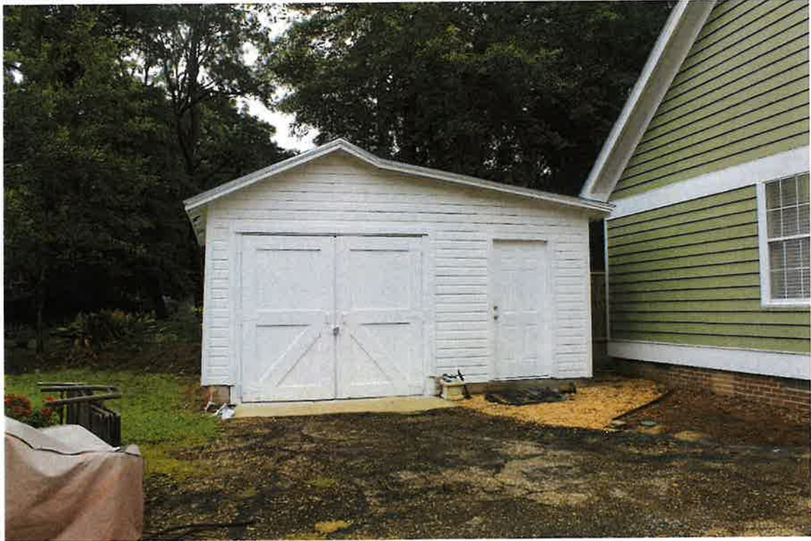
660 Cloverdale Road (Old Cloverdale), view to rear yard and detail of garage, 06/05/2024
