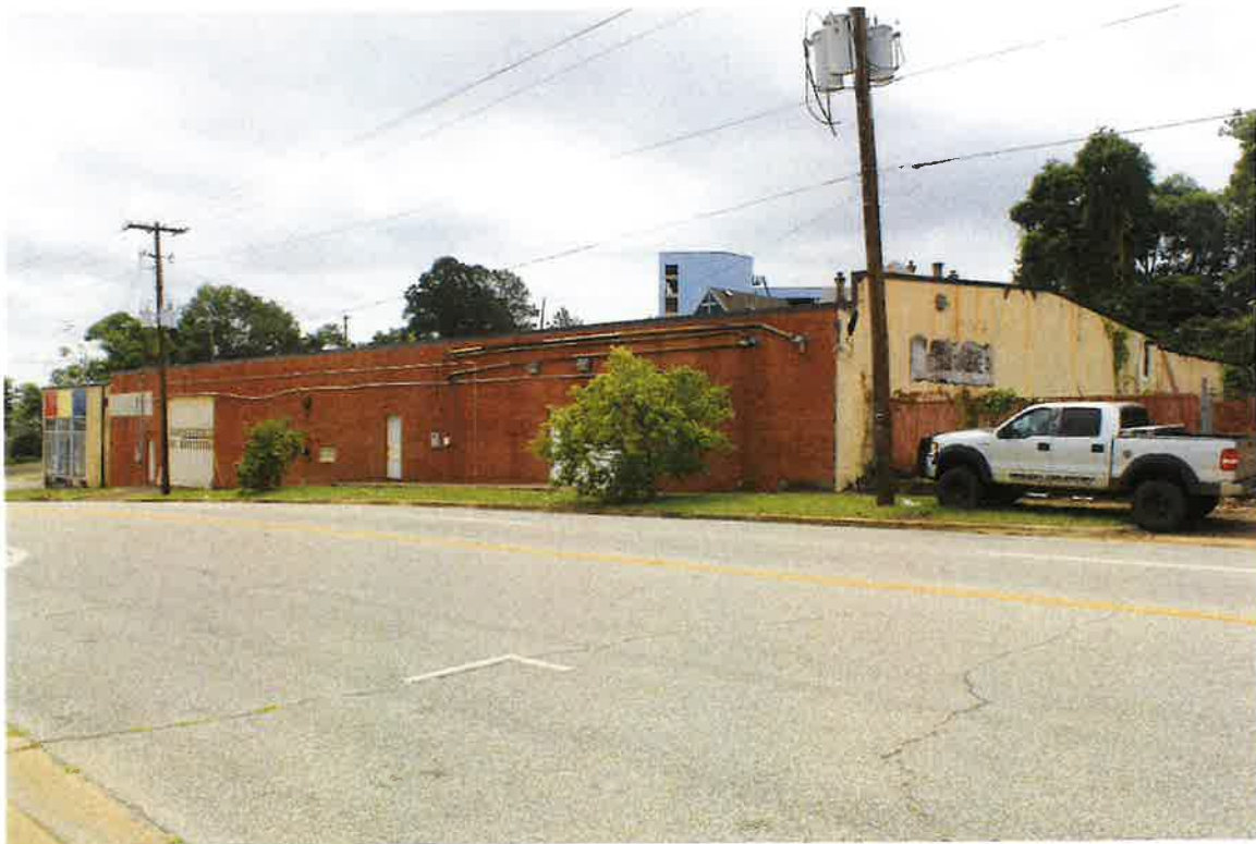
121 N. Goldthwaite Street (Cottage Hill), east façade and north elevation, 06/05/2024
