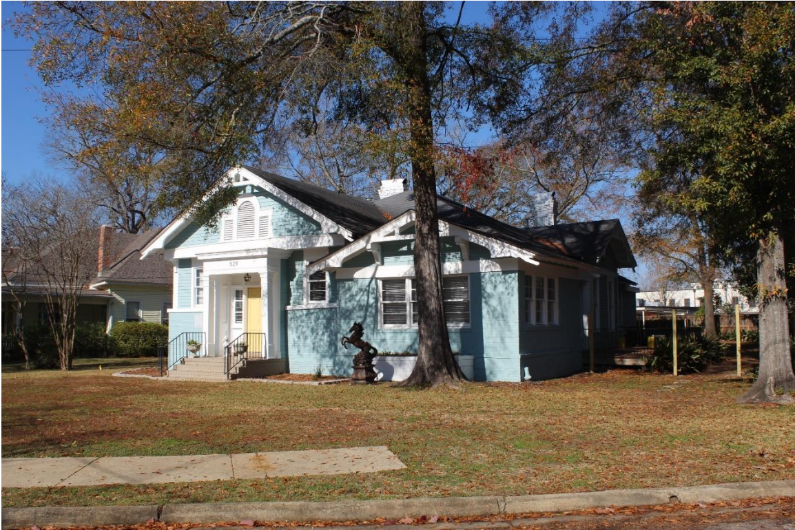
Figure 17: 529 Felder Ave, south façade, and east elevation, facing northwest
