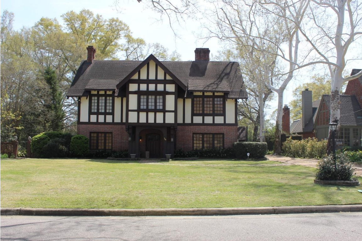
Figure 21: 728 Thorn Place, north façade, 03/14/2024
