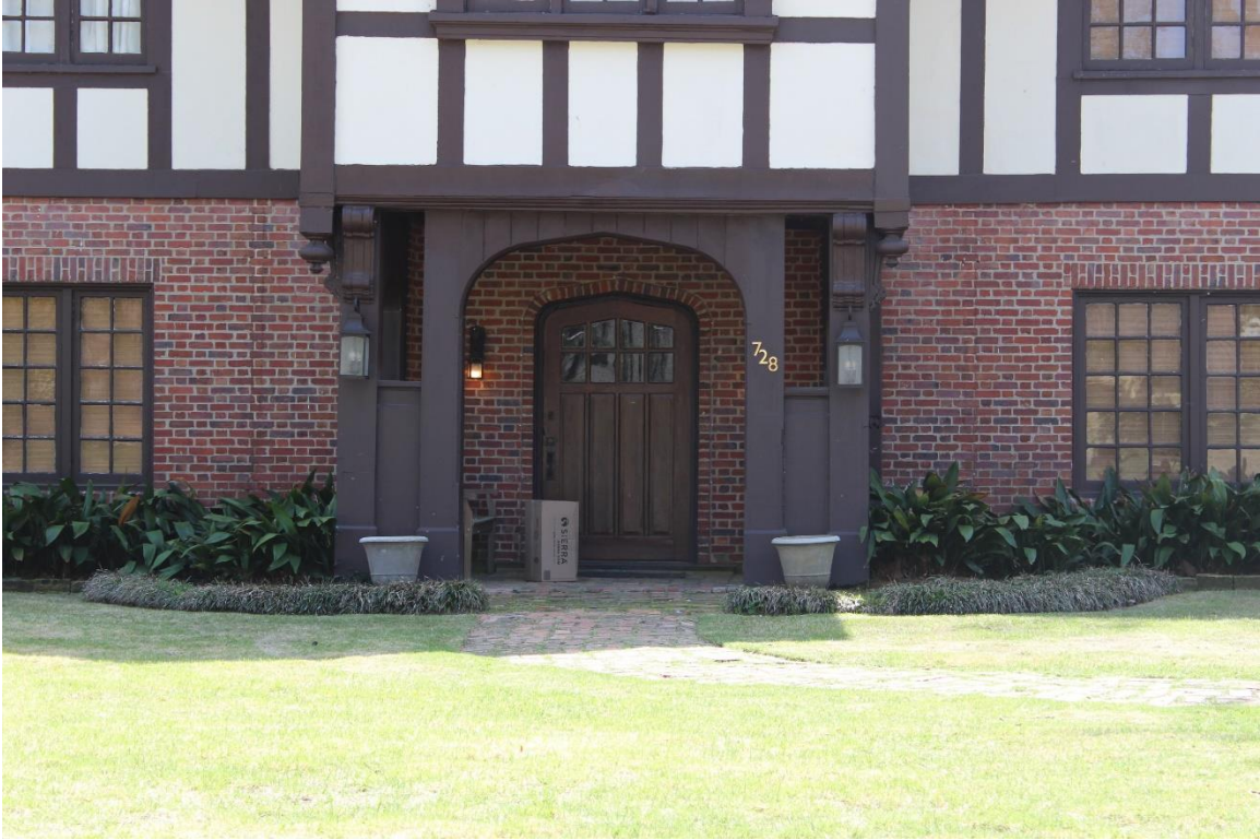
Figure 23: 728 Thorn Pl, main entry door detail, 03/14/2024
