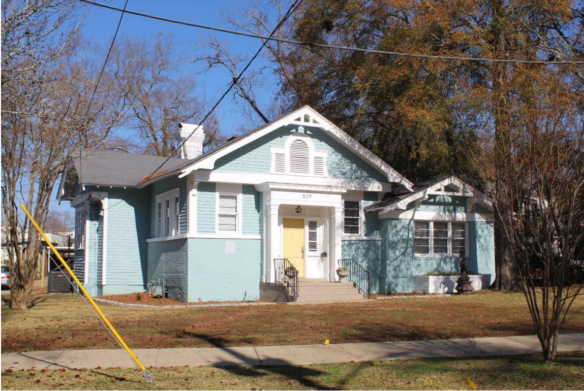
Figure 16: 529 Felder Ave, west elevation, and south façade
