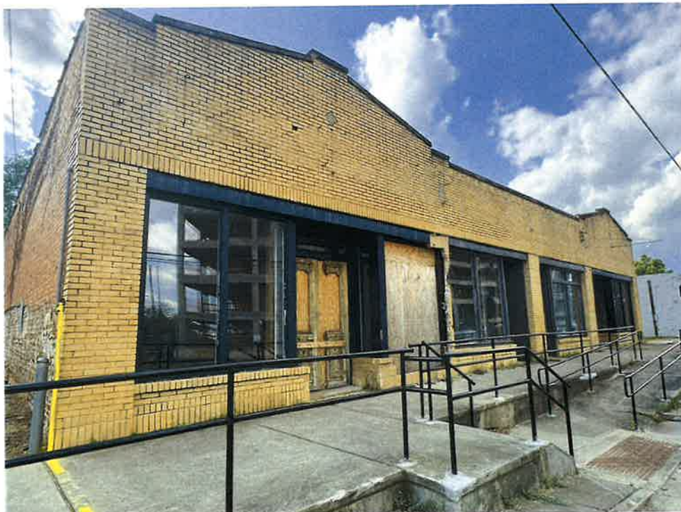
Existing building front (east elevation)
