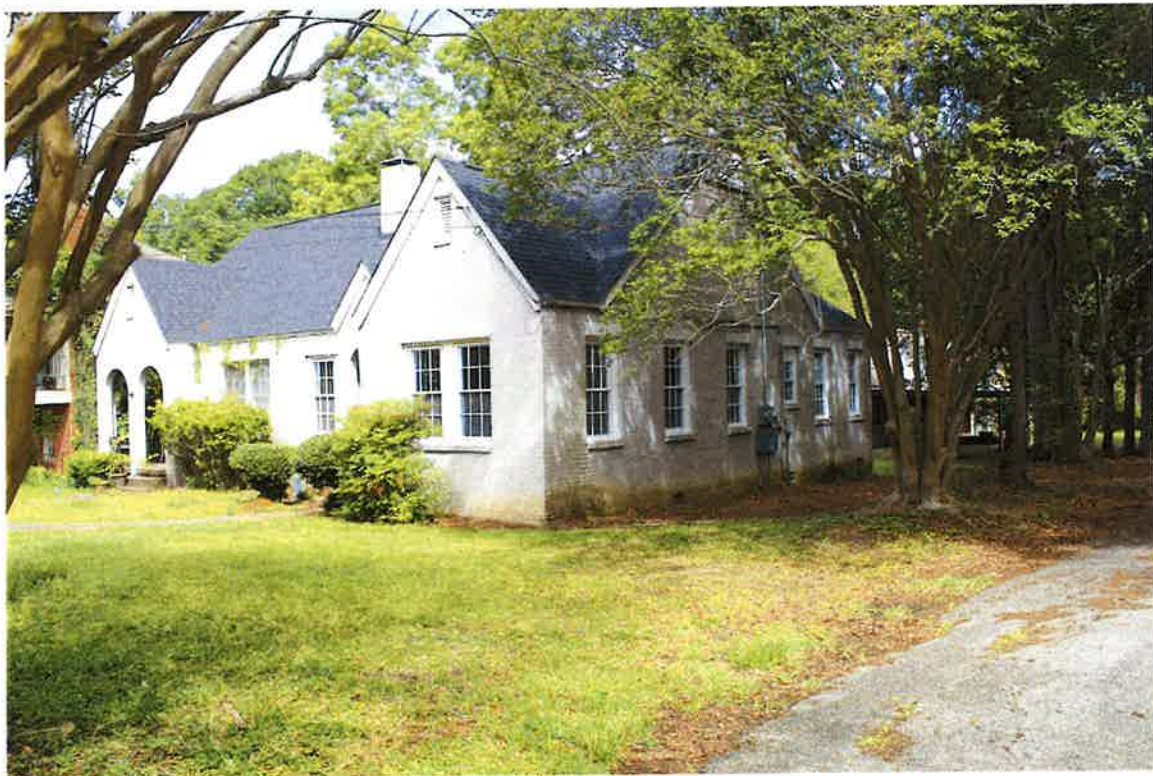
1131 Magnolia Curve (Old Cloverdale), current condition with replacement windows, 04/10/2023
