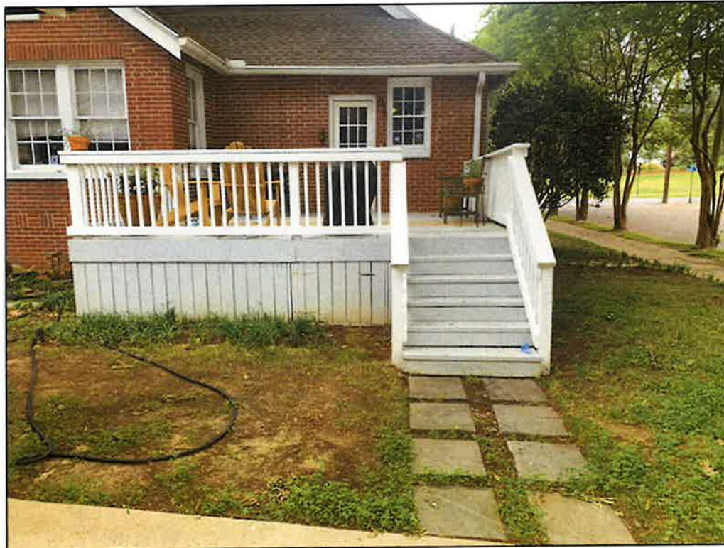
303 Felder Ave (Garden District), North (rear) elevations with view of deck, 04/16/24
