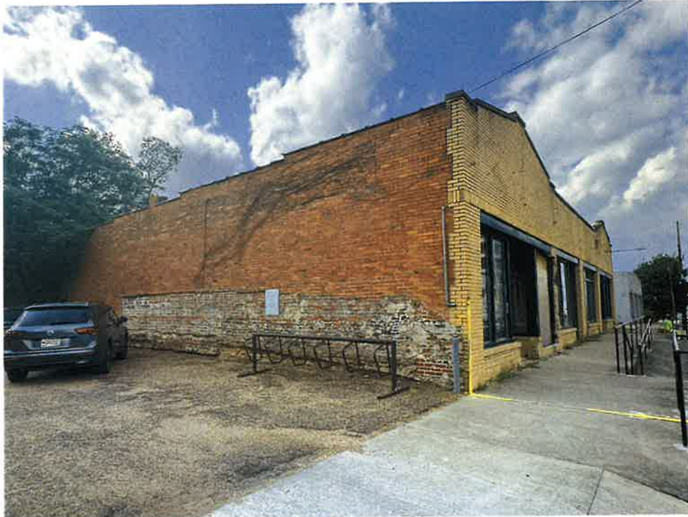
Existing building (south elevation)
