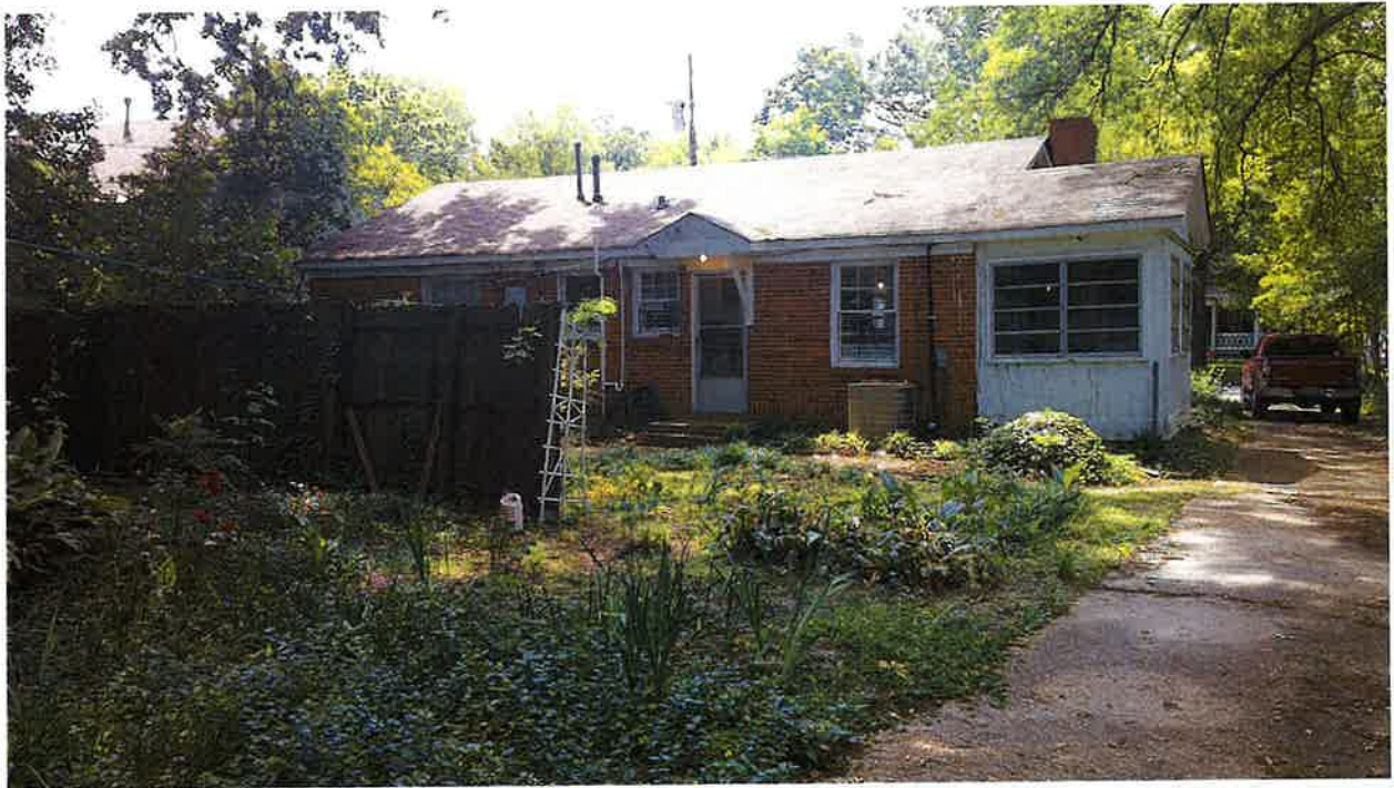
1924 Norman Bridge Court, Garden District, north and west elevation of outbuilding with detail of deterioration; north (rear) elevation of main residence
