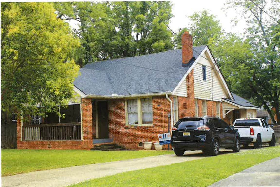
3124 Lexington Road, Cloverdale Idlewild, east façade, and north elevation, 05/10/24
