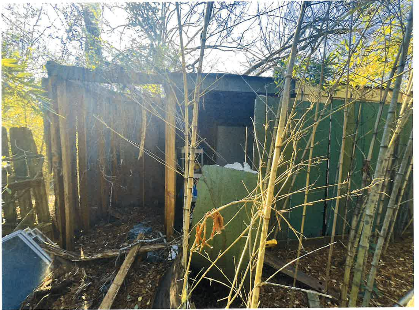
Shed for demolition
