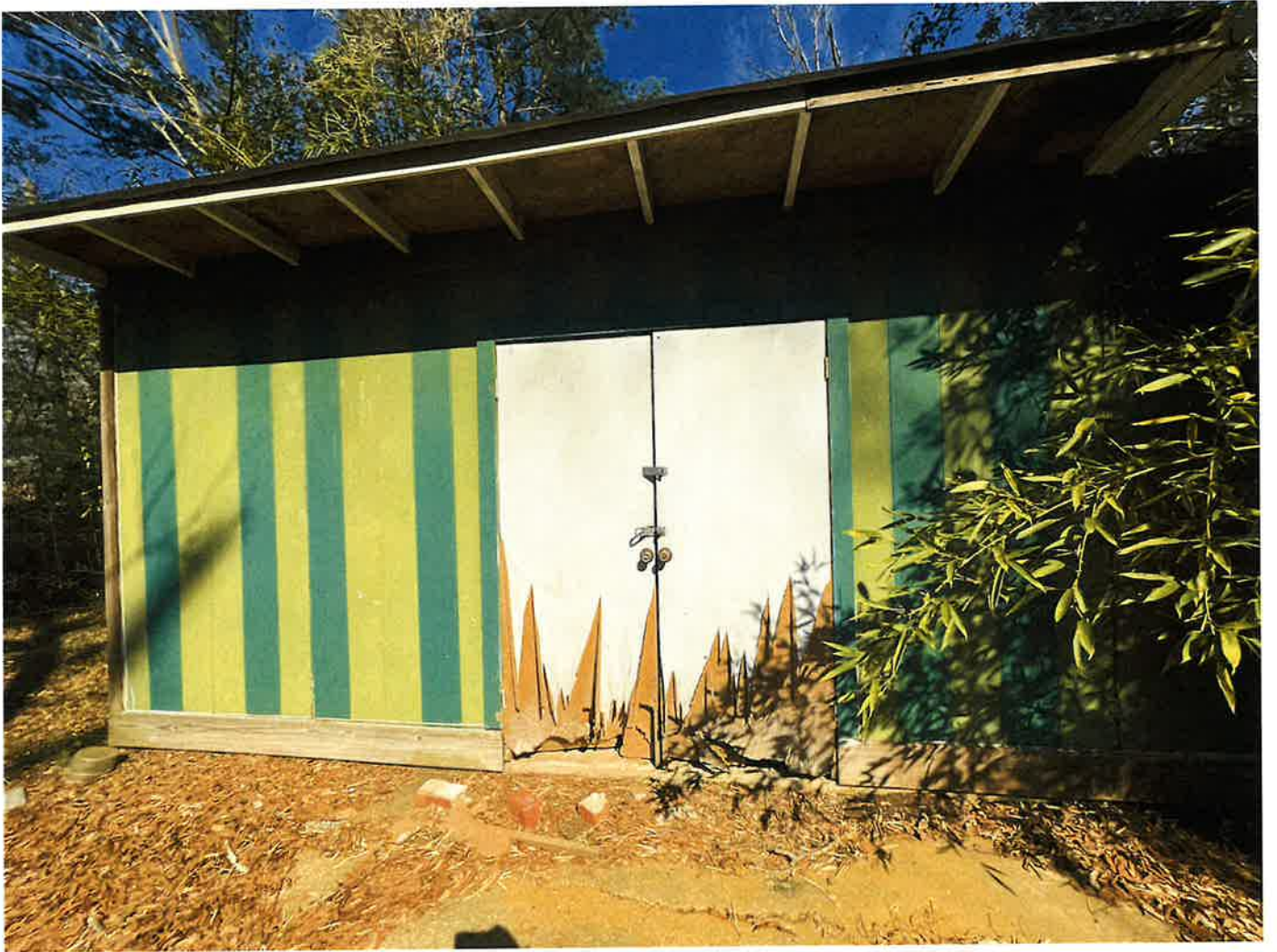
Shed for demolition
