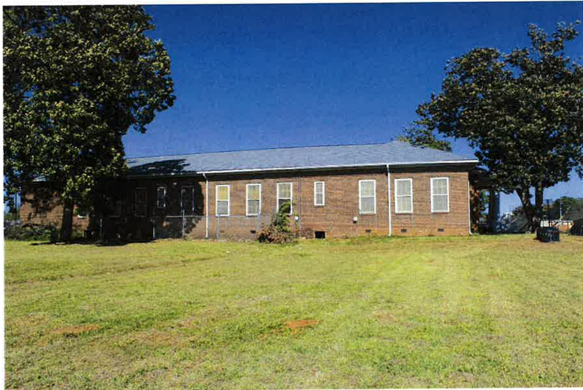
1020 Maxwell Boulevard (Individual Designation), south façade and west elevation, 04/04/24
