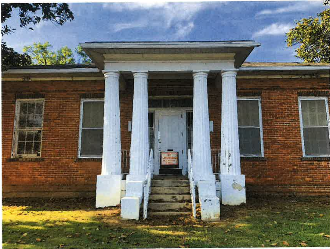
1020 Maxwell Boulevard (Individual Designation), south façade context and detail, 03/28/24, 04/04/24
