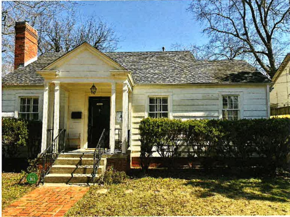
1. 1909 Graham Street - Front facade (west)
