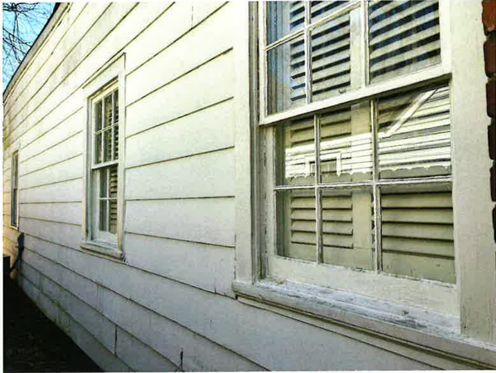
3. 1909 Graham Street - North side 2 of 2
