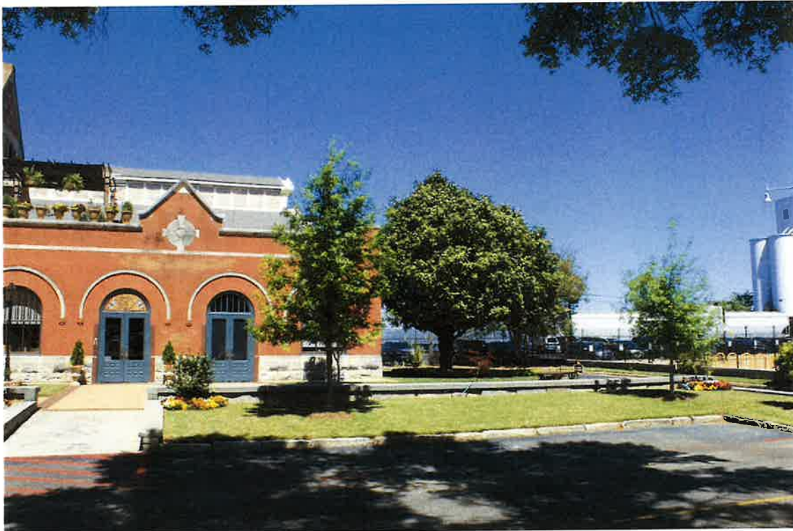
210 Water Street, Lower Commerce, south façade, and view to project area, 04/04/24
