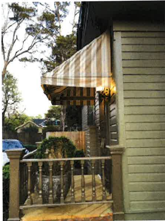
2203 Felder Terrace, Old Cloverdale, current fabric awning, 03/28/24
