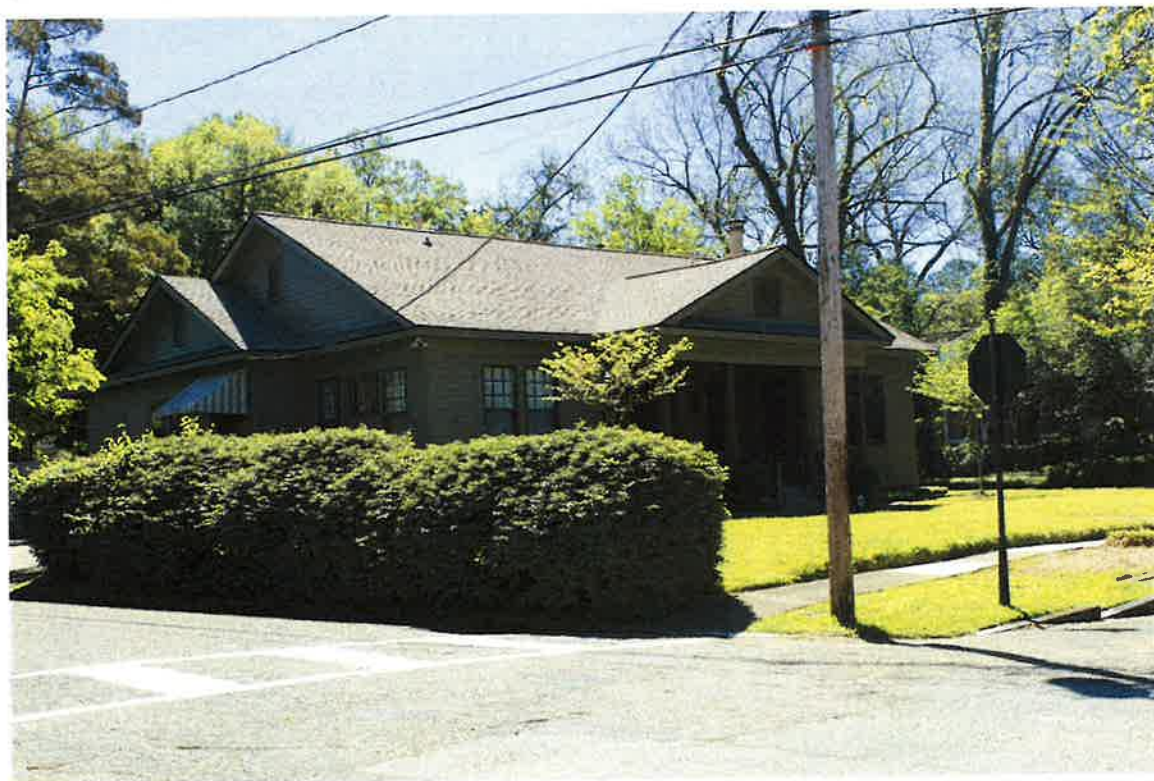
2203 Felder Terrace, Old Cloverdale, East façade, and North elevation, 04/04/24
