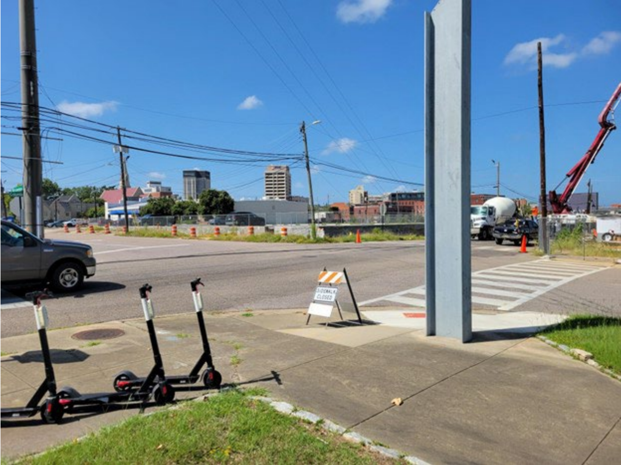
Photograph 3: Hotel construction west of MW-085
