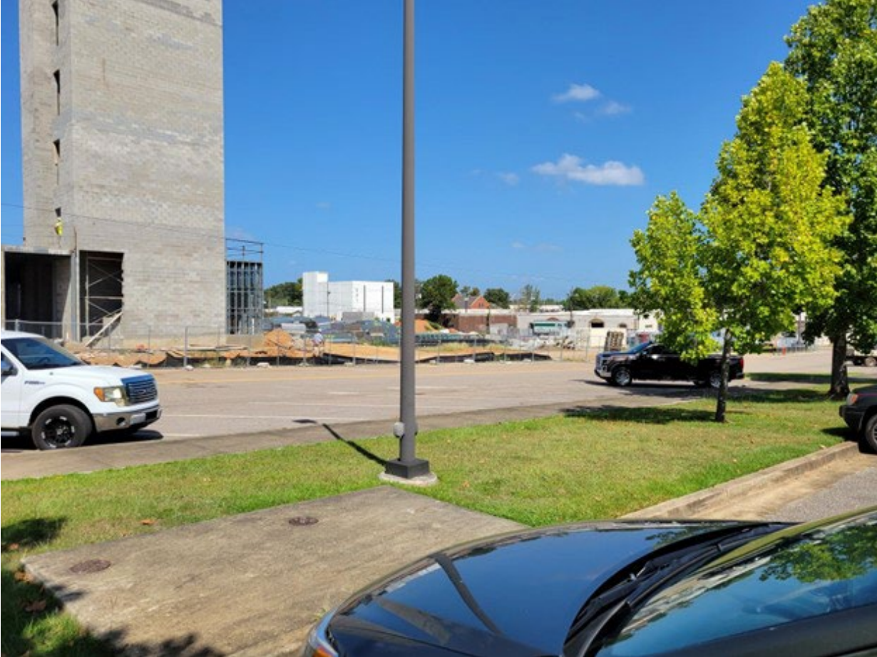
Photograph 4: Hotel construction west of MW-08S
