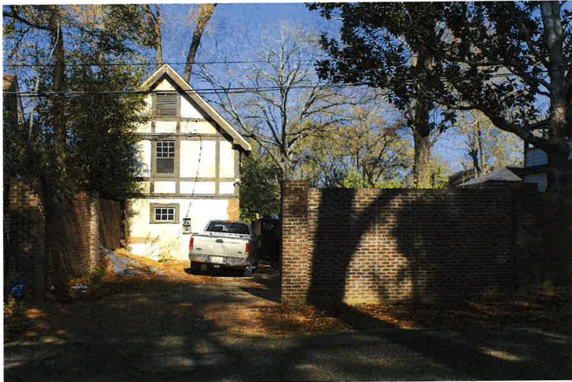
1324 S. Perry Street, Garden District, west elevation (rear) context and wall, 01/04/24
