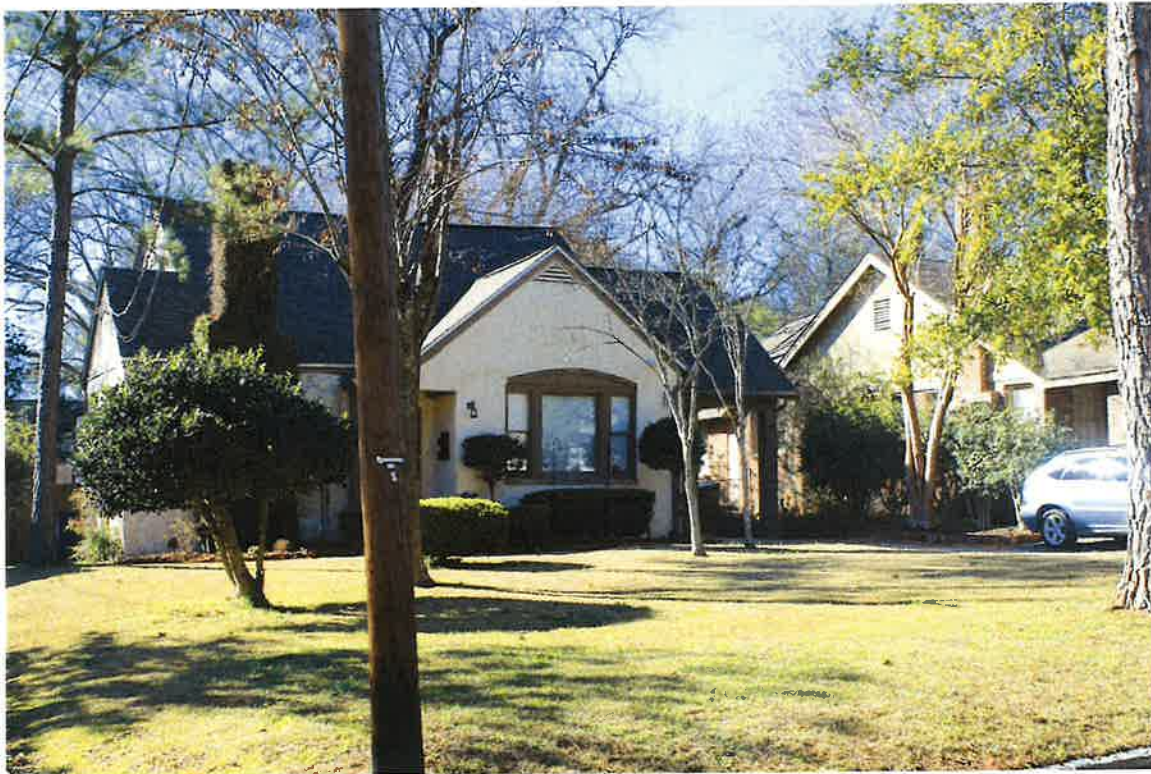
3360 Montezuma Road, Cloverdale-Idlewild, east façade and subject tree (at right), 02/13/24
