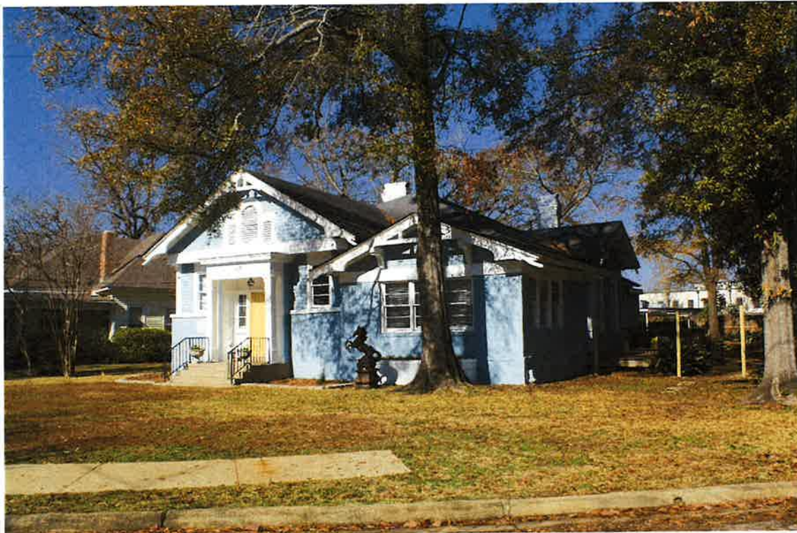
529 Felder Avenue, Old Cloverdale, South façade, west and east elevations, 01/04/24
