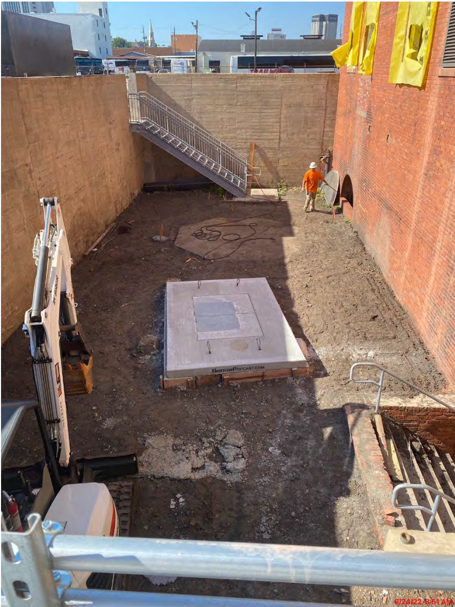
608 North Court Street – Capped Pit
