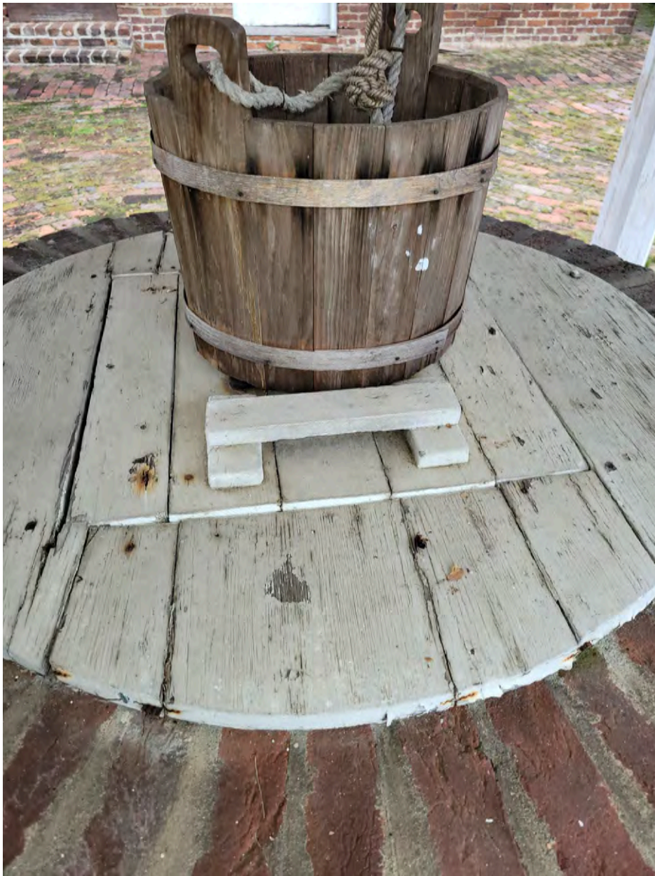
230 North Hull Street – Historical Bucket Well, Secured Lid
