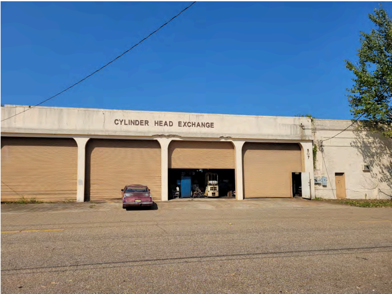
507 North Perry Street
