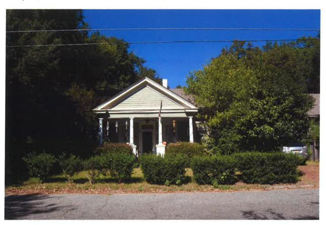
One story gable on hip bungalow; front gable projection over porch supported by groupings of 3 square columns on brick piers at corners and not intermediate supports; open fretwork and engaged brackets one ends of house with ogee arches(similar to 419 Clanton); tripartite gable combo of 6 lite window flanked by 2 louvered vents; 12:1 and 9:1 wood windows; decorative eave brackets in all gables; wood siding on front elevation, vinyl on sides. Original full lite front door with 3 lite transom. C
