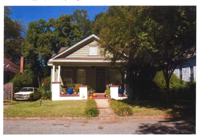
One story Folk Victorian pyramidal roof with asymmetrical front gable projection with pent roof; screened shed roof porch tucked into projection; triple hung block pattern oversized window; 2:2 wood windows; vertical 3 lite half glass front door with 2 lite transom. C
