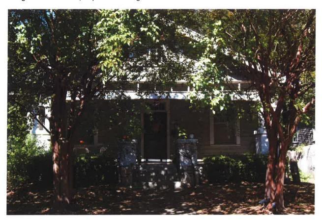
One story hipped roof Folk Victorian with hipped roof porch supported by newer metal columns on brick piers; 4:4 wood windows; two lite front door with arched glass panels and sidelights appear to be from an older house (details on surround more typical of Greek Revival or Italianate); wood siding; replacement porch rail. C
