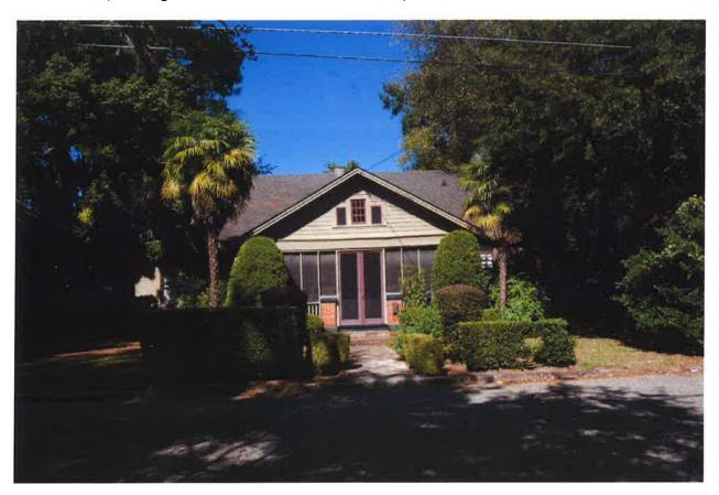
One story cross gable bungalow with Classical Revival details; gables are pedimented with partial cornice returns and sheathed in wood shakes; wood drop siding; porch supported by round Tuscan columns on brick piers; ¾ wood front door with one lite transom; 9:1 wood windows. C
