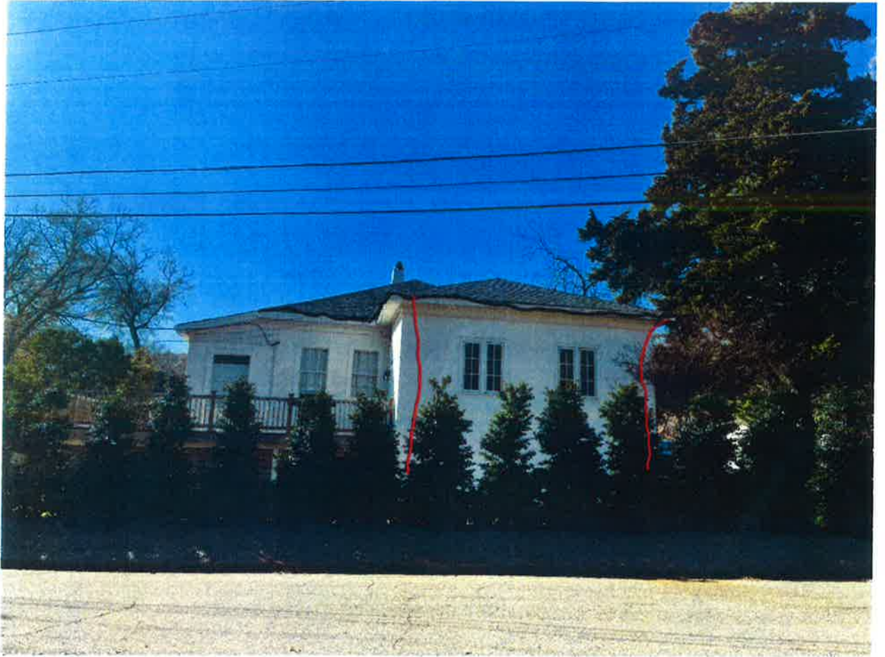
4. Comparable homes within ½ mile with similar non-intrusive drainage systems.
