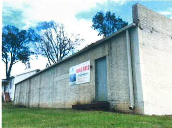
SIDE VIEW (West)
