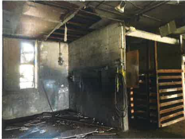
INTERIOR – THIRD WAREHOUSE (North)
