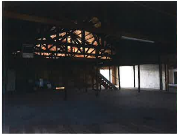
INTERIOR – FOURTH WAREHOUSE (East)
