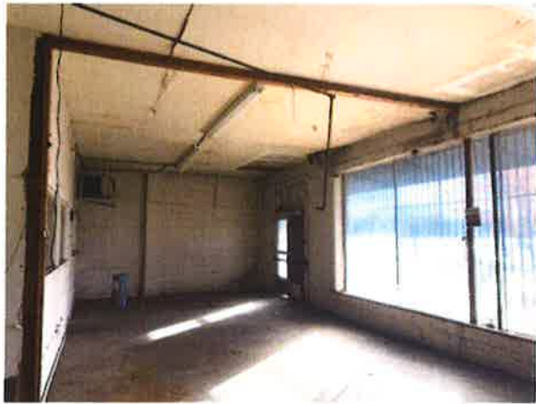
INTERIOR - FIFTH WAREHOUSE (East)
