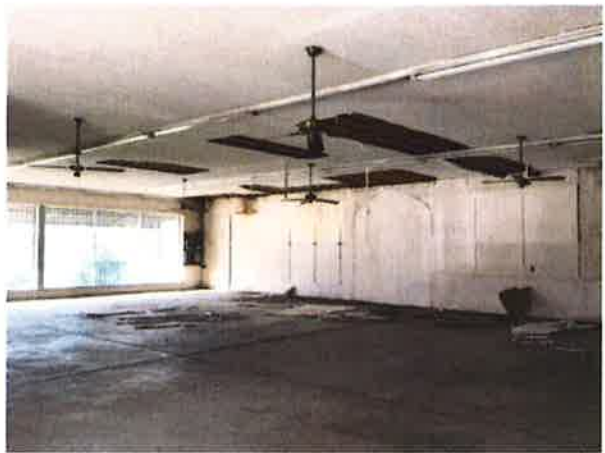
INTERIOR – FIRST WAREHOUSE (South)
