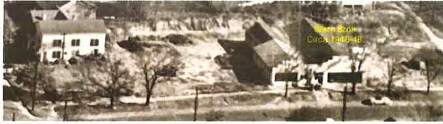
ORIGINAL STRUCTURE (Circa 1946-1948)
