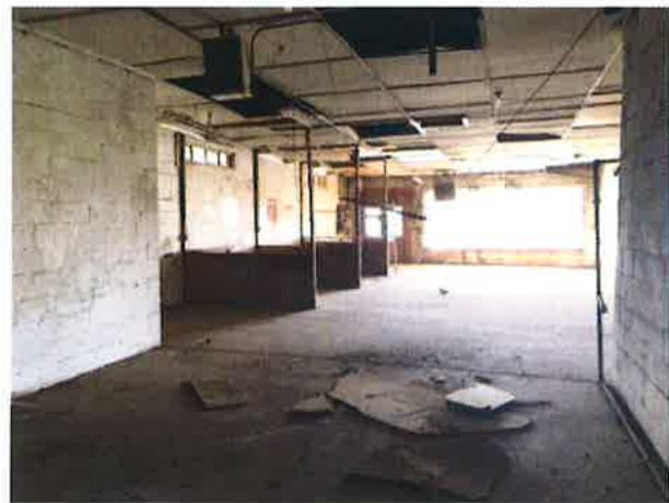
INTERIOR – THIRD WAREHOUSE (South)
