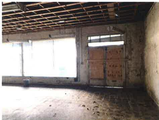
INTERIOR – FOURTH WAREHOUSE (South)
