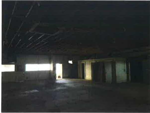
INTERIOR – FIFTH WAREHOUSE (South)
