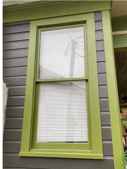
Window stripped, oiled, relglazed and repainted
