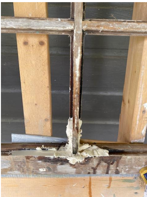
Filling with wood epoxy
