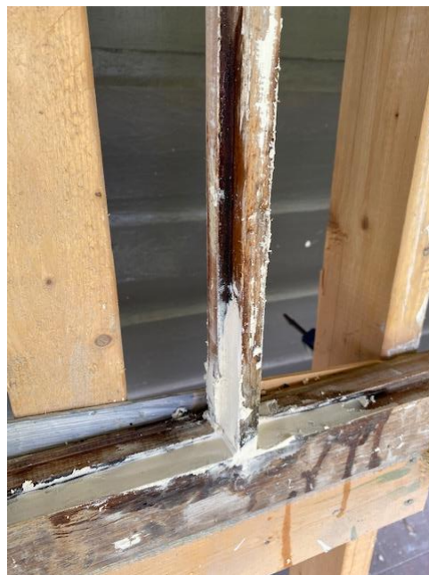
Epoxy tooled to window shape before sanding
