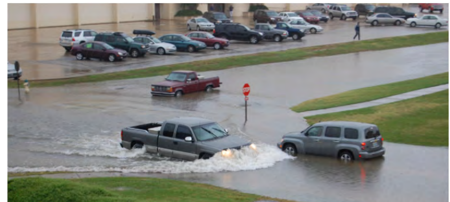
Base flooding during major rain events. Photo credit: Carl Bergquist
