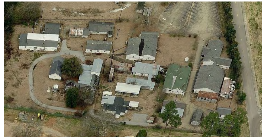
State-owned property with abandoned structures
