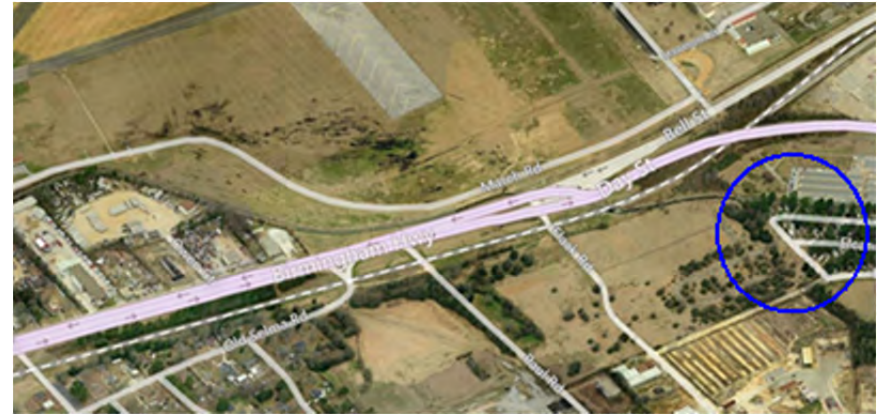
Aerial of Maxwell AFB Runway 33 Clear Zone and Trees
