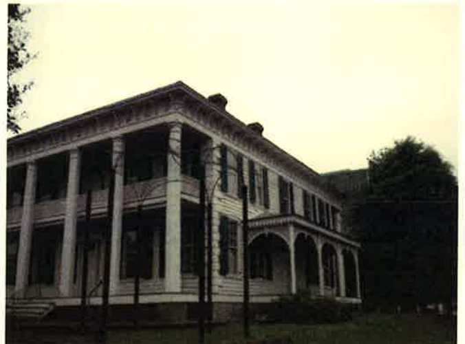
West side with metal porch roof to be replaced with like material
