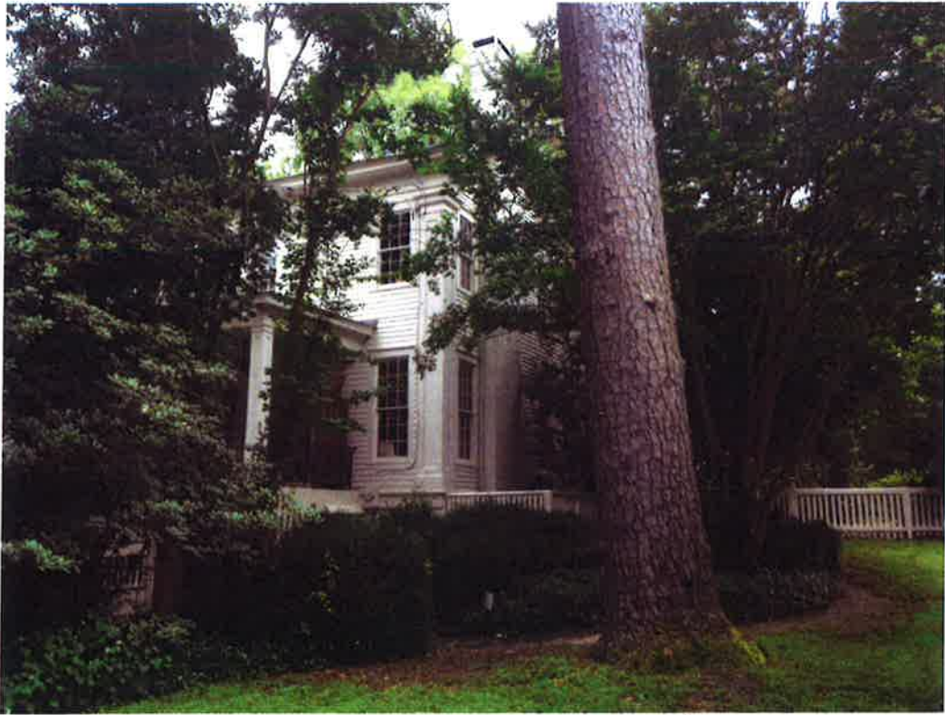
Side rear view where the proposed addition would be located
