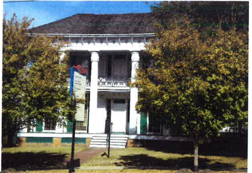
Overall front/south view of existing wood shingles to be replaced with architectural tab shingles
