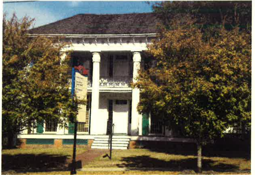
Overall front/south view of existing wood shingles to be replaced with architectural tab shingles
