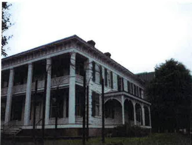
West side with metal porch roof to be replaced with like material
