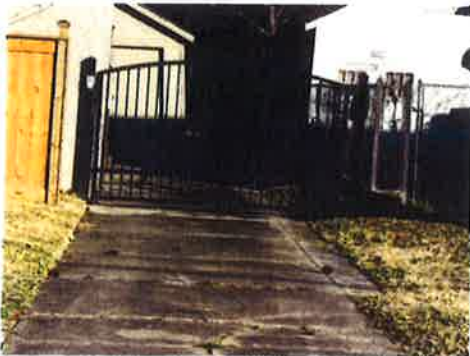
Neighbor's gate also installed by A+. 3317 Montezuma Rd
