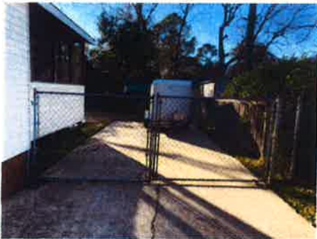
Chain-link gate to be replaced
