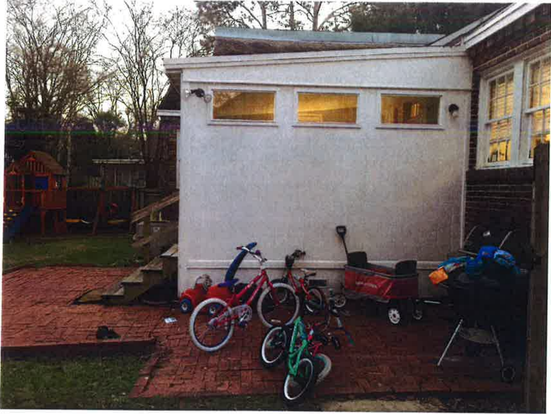
Project 1: Existing North Elevation (Side of House)
