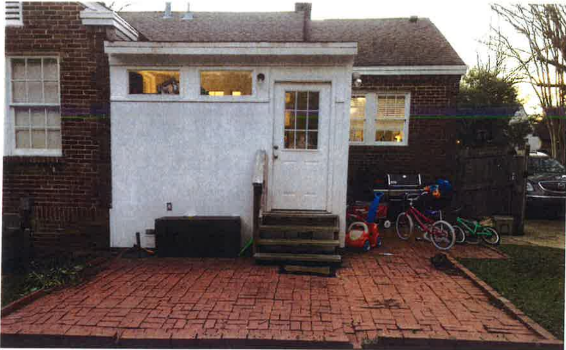
Project 1: Existing East Elevation (Back of House)
