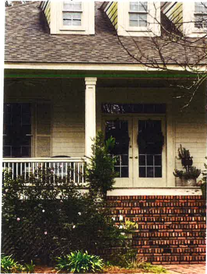
15. Close up of square colonial columns at 2401 E Cloverdale Park.
