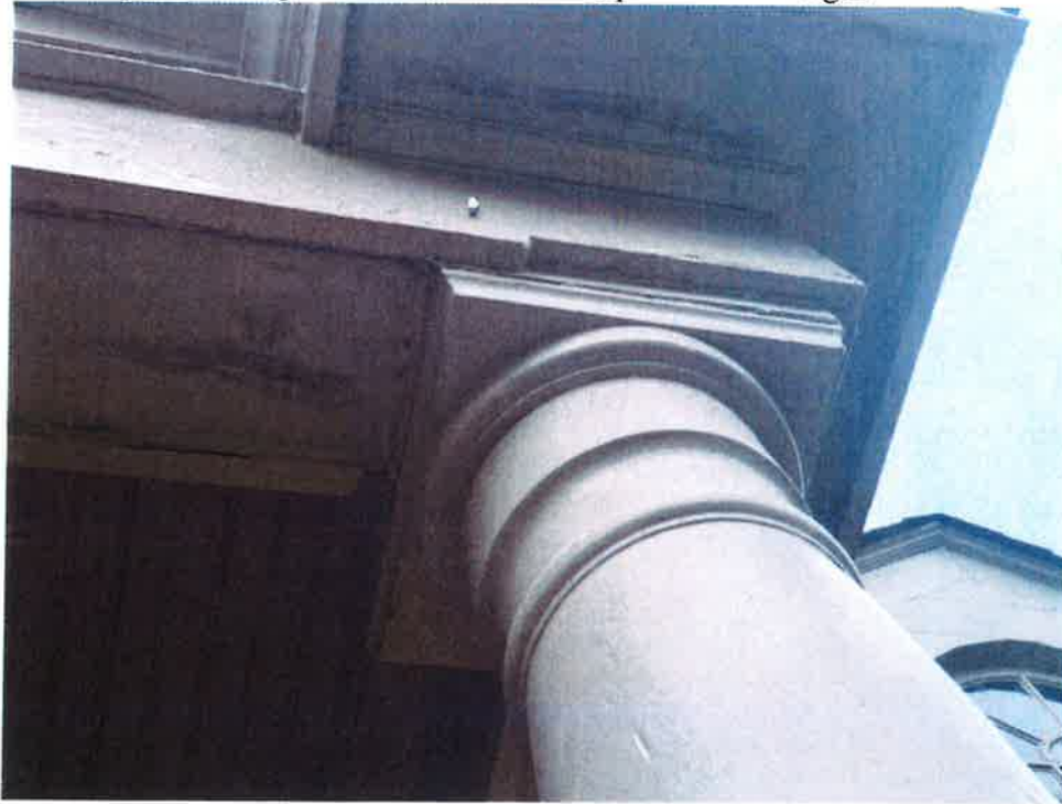
6. Disruption to original woodwork at the top of the front right column.
