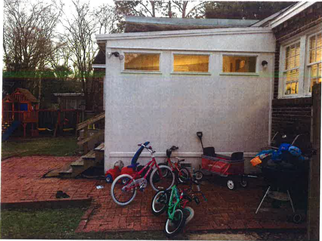
Project 1: Existing North Elevation (Side of House)
