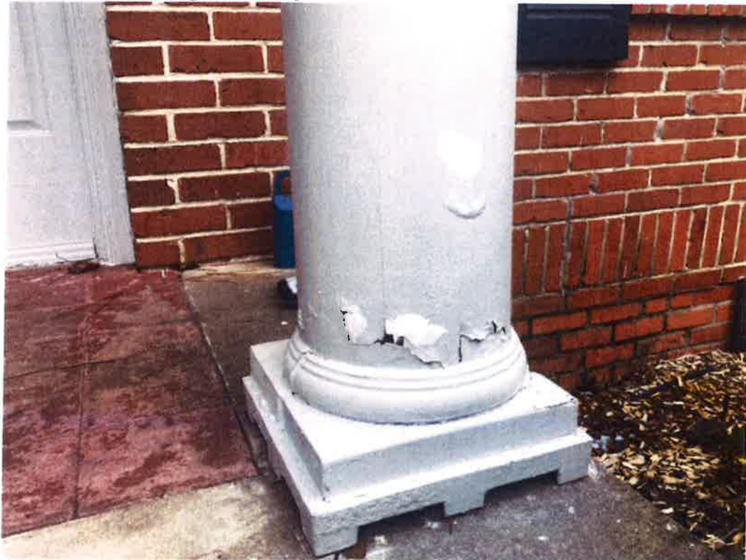
4. Evidence of rotting of front right column.
