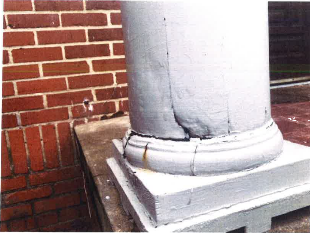
4. Evidence of rotting of front right column.
