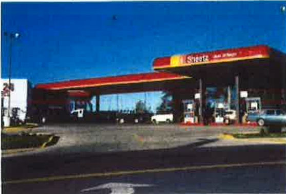
Typical new service station
