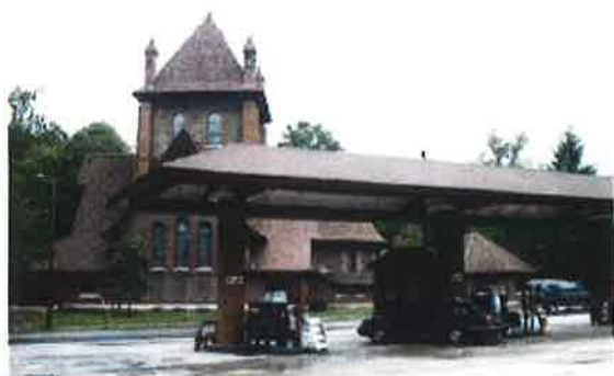
BP Station in Asheville, North Carolina, shows that gas station canopies can come in all sizes and shapes.
