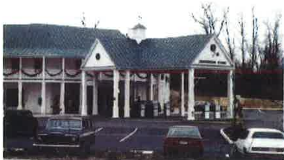
New service station, Albemarle County, Virginia, has a standing seam metal roof like other nearby buildings.
