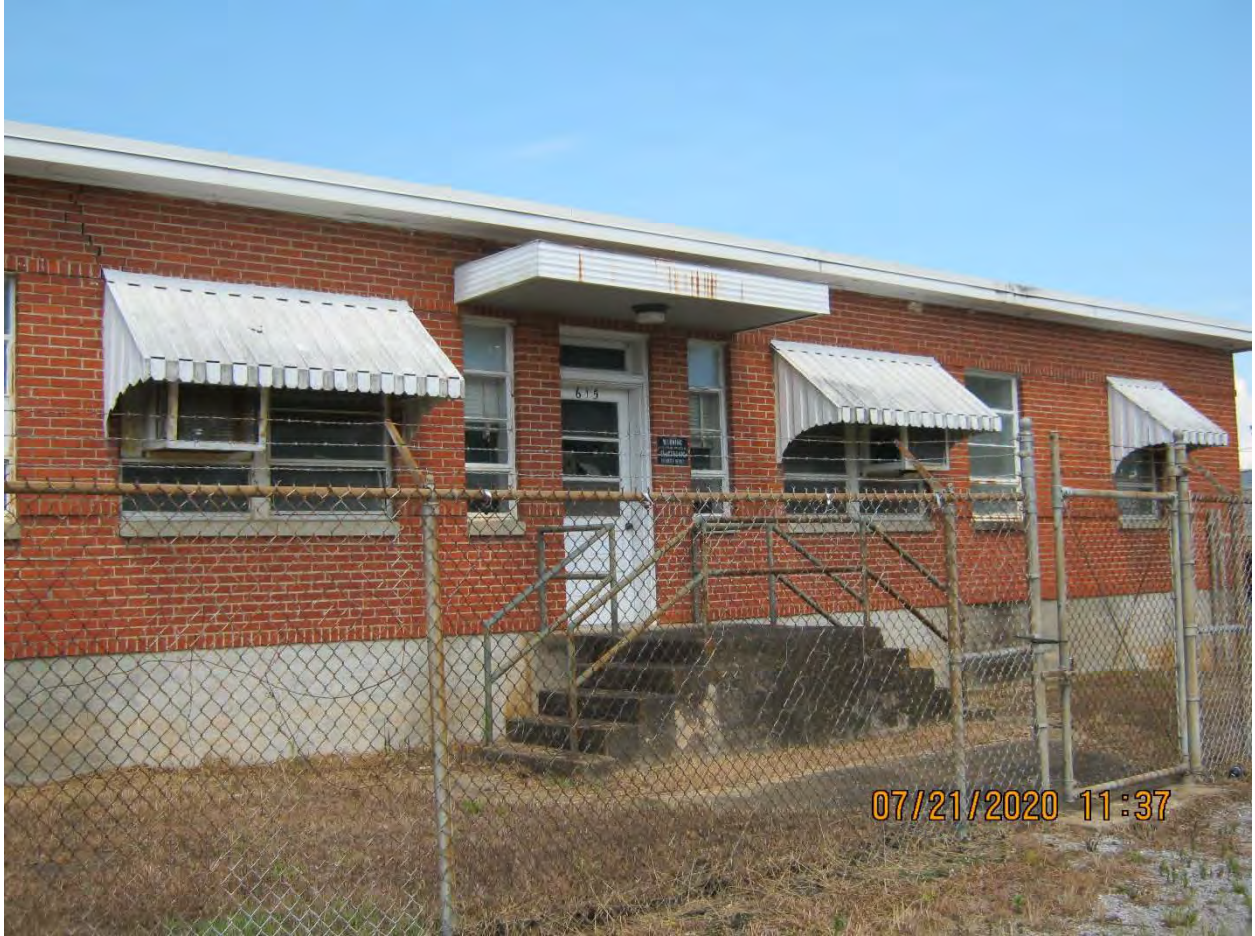
615 North Perry Street
