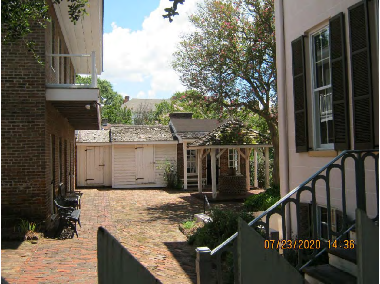
230 North Hull Street
