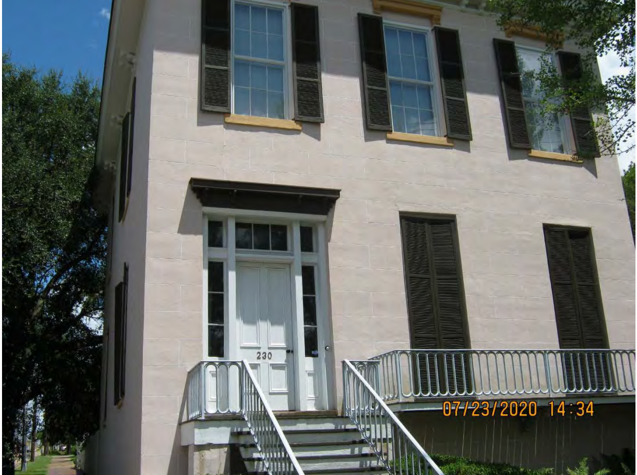
230 North Hull Street
