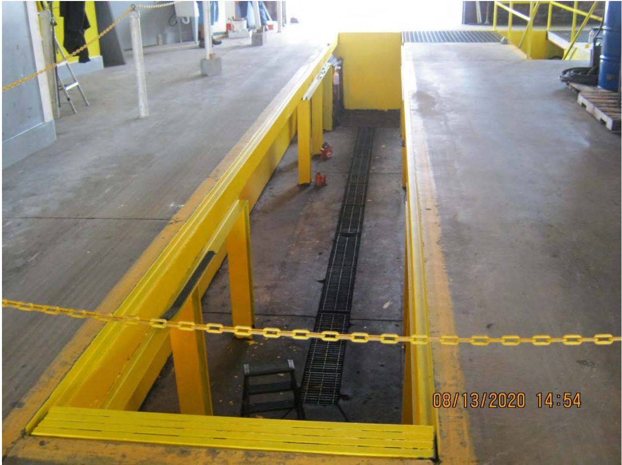
520 North Court Street
