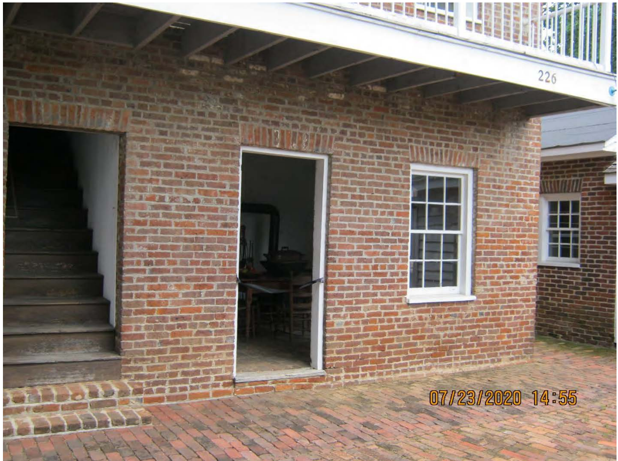
230 North Hull Street
