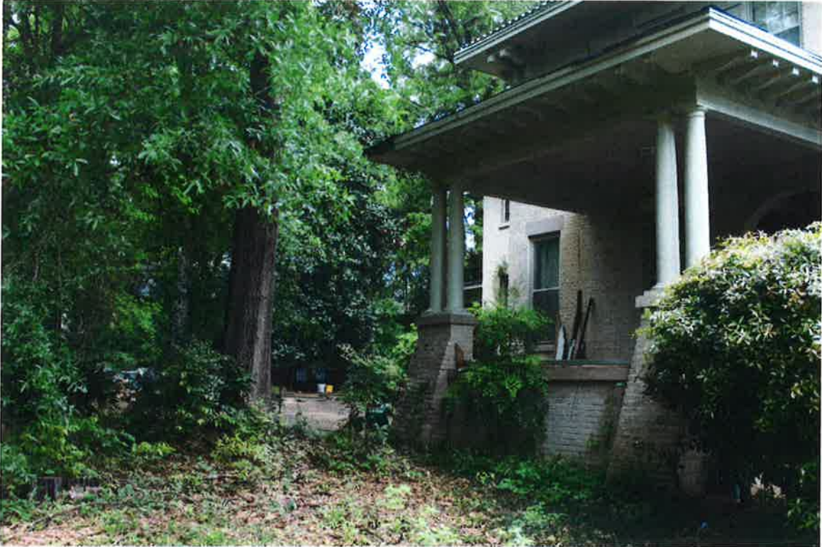
Back of porte cochere
