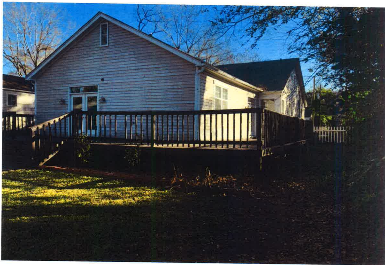
1910 Graham Street Rear View with Deck
