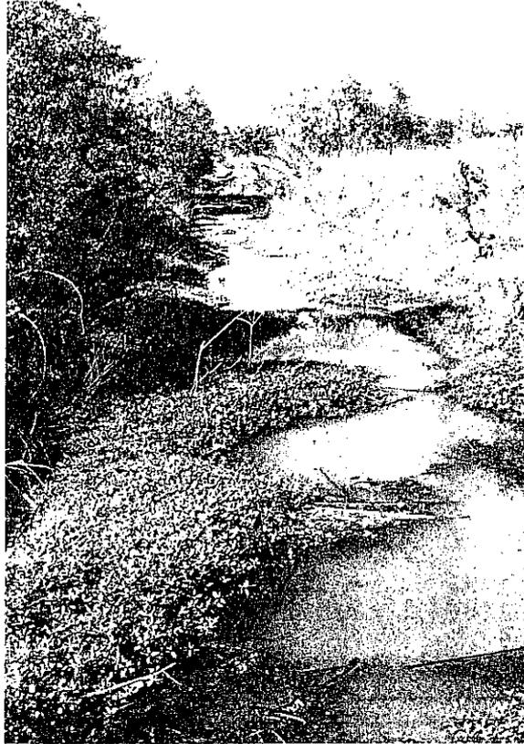
FIGURE 2-13. Poor channel conditions downstream of Terminal Road Culvert cause standing water and dense vegetation.
