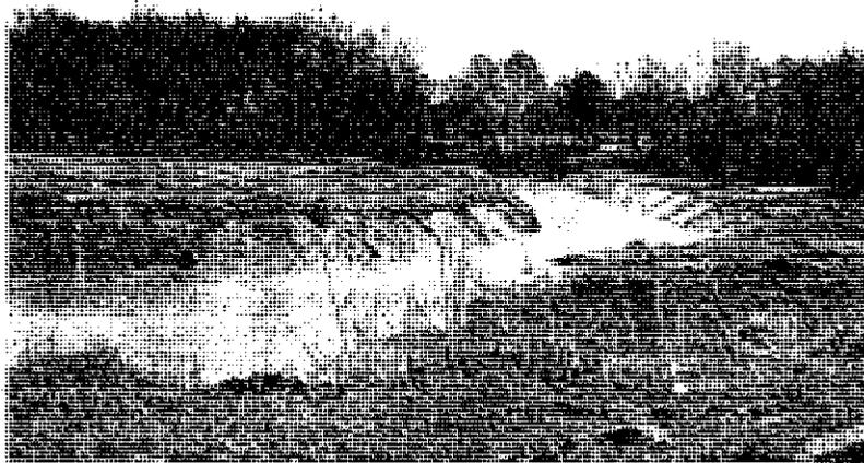
FIGURE 2-4. Concrete-lined open channel at the confluence of Sherwood Ditch and Three-Mile Branch.
