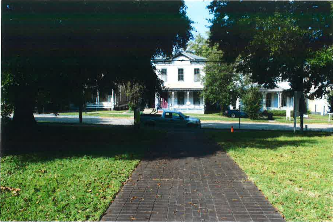
View looking toward street to show grade change at ROW
