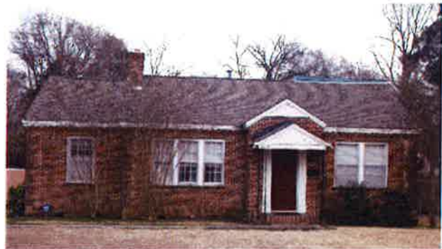
Front elevation showing painted brick. (Current)
