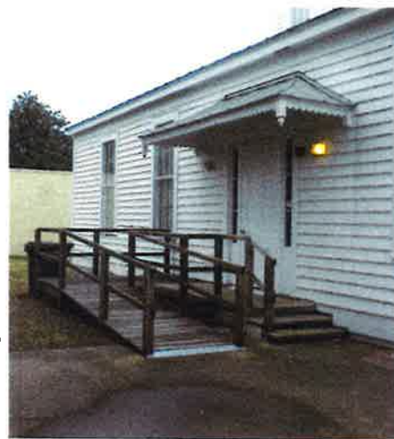
ADA access requirements are met on the rear of the building with existing ramp.
