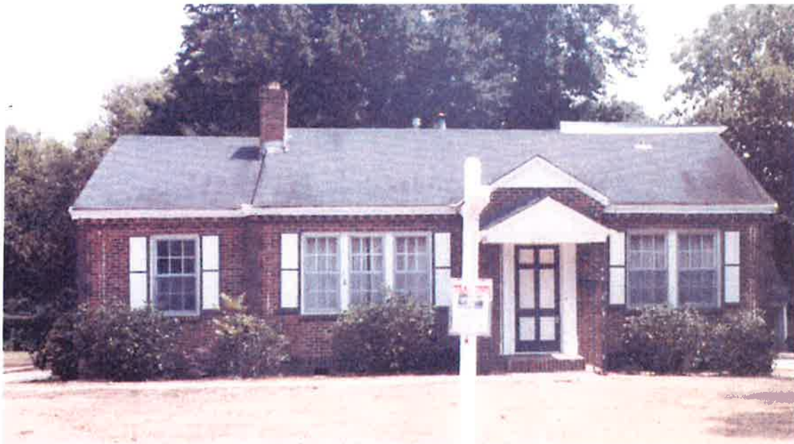
Front elevation showing shutters and course of painted brick. (Historic district survey)
