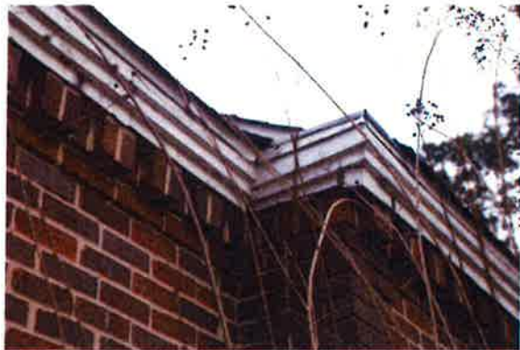
Fascia with painted brick
