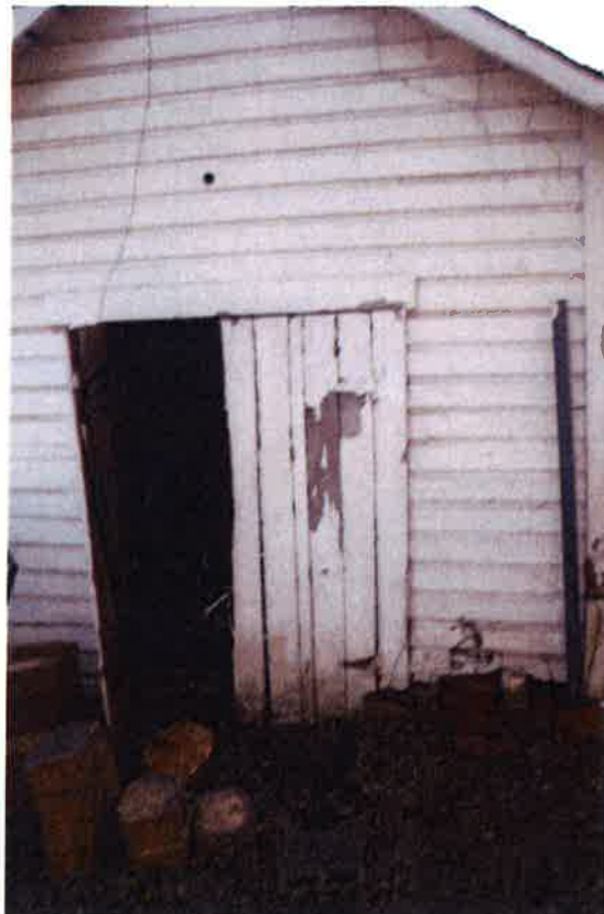
Rear opening to be closed
