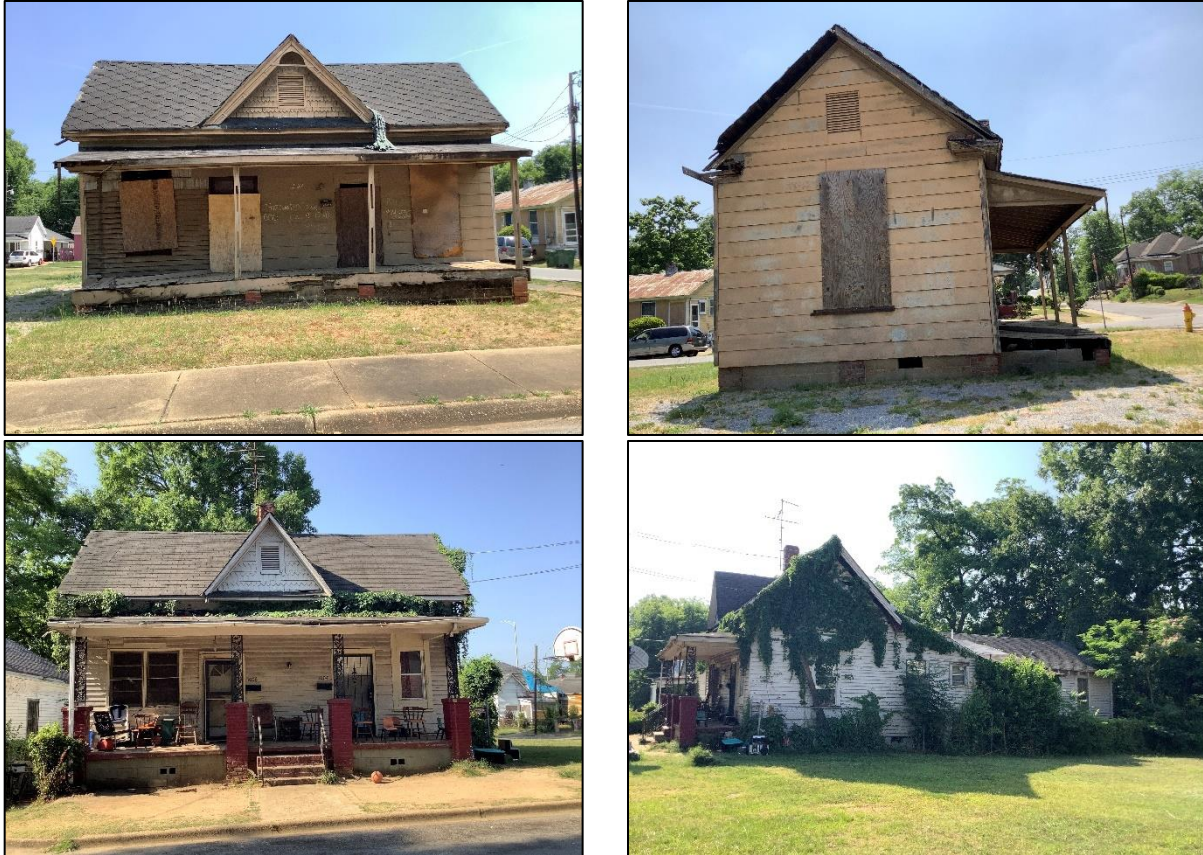
Figure 2. Two-room Victorian-style homes in Centennial Hill. Top: the only remaining example with no additions. Bottom: an example of common alterations and additions for this type of home.
