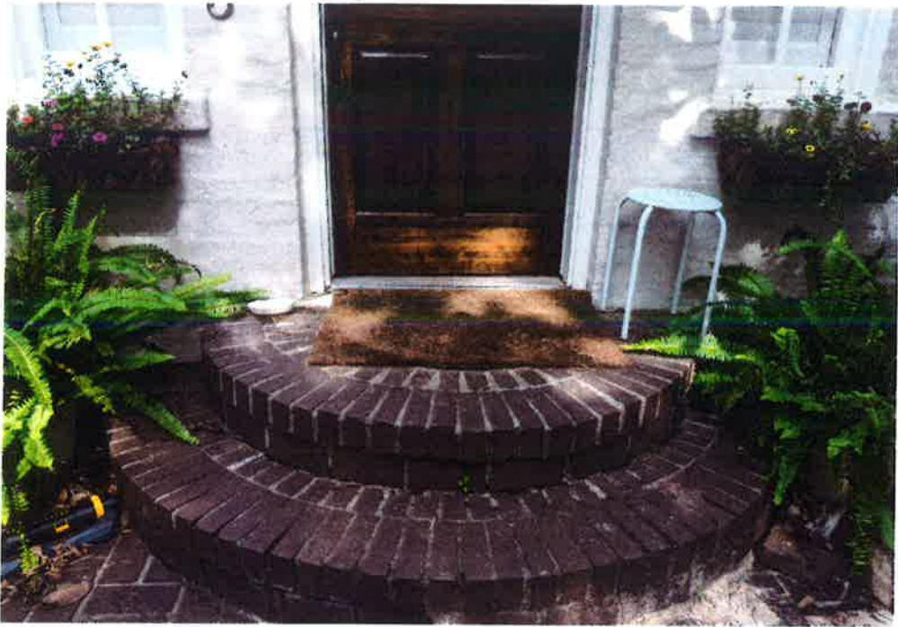
Existing Brick Stoop
